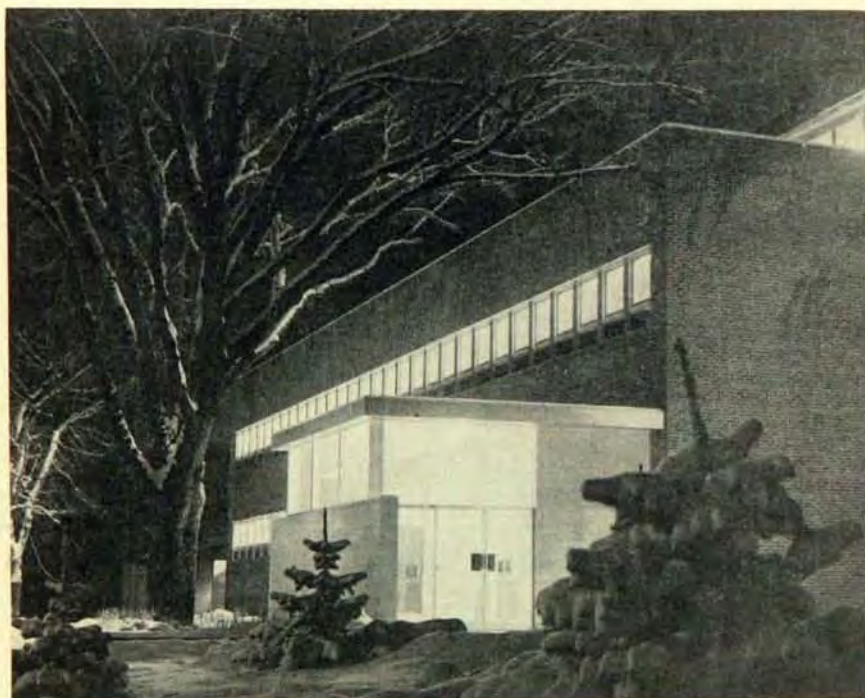
NEW BUILDING ON ST. PAUL CAMPUS
