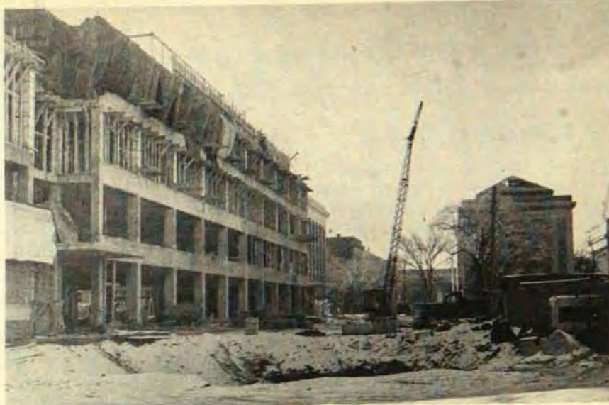
The new Mechanical-Aeronautical Engineering building which adjoins the Electrical building will be completed this coming spring. The new building faces the Administration building which is shown in the background.
