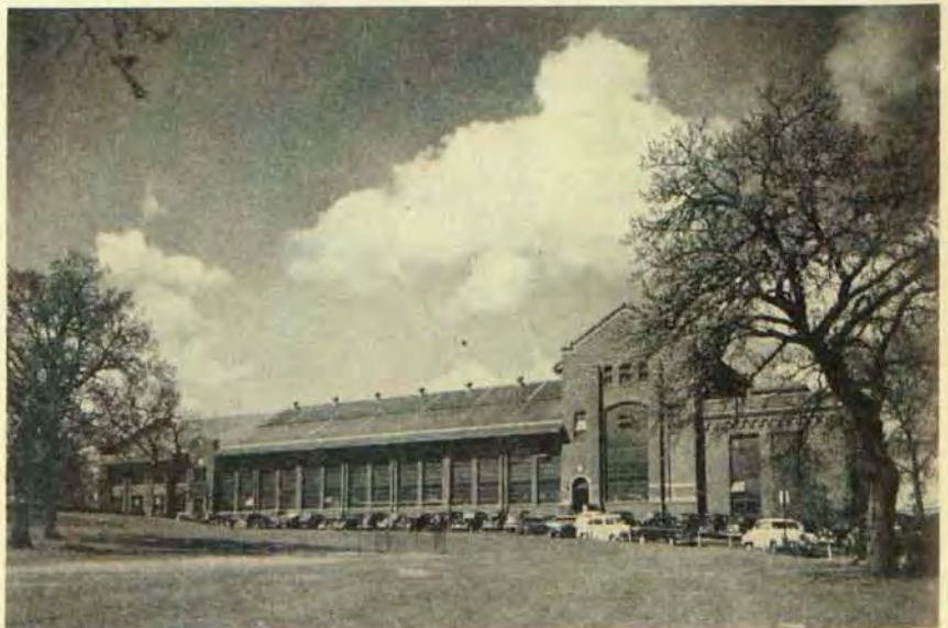
Mines Experiment Station on the Minneapolis campus of the University of Minnesota.
