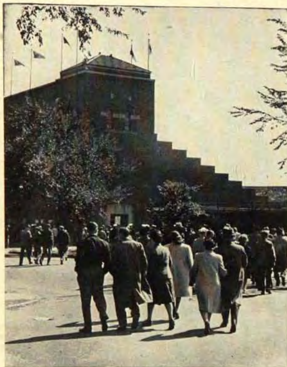
North Tower, Memorial Stadium
