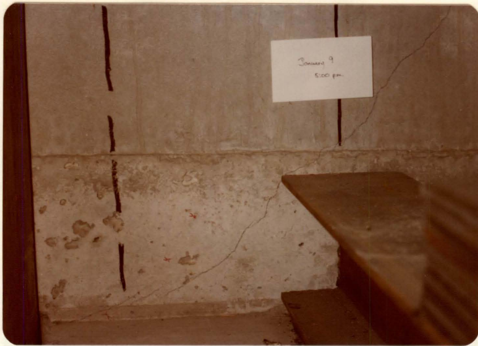
Photograph #13 - Front-View Stem, Displaying Diagonal Hairline Crack at Load Stage #4. (North-End Reaction)
