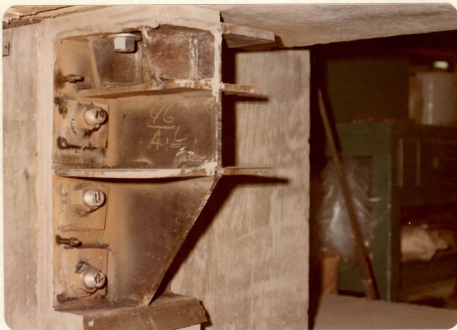
Photograph #10 - Side-View of Steel Haunch After Grout was Installed. (South-End Reaction)
