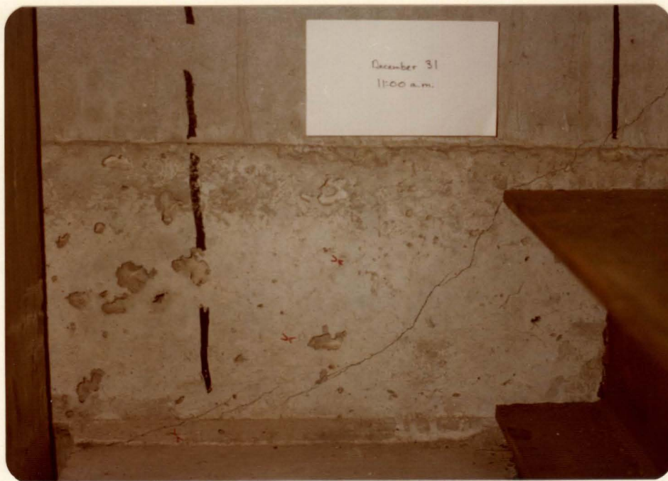
Photograph #14 - Front-View of Stem, displaying Diagonal Hairline Crack at Load Stage #4. (North-End Reaction)
