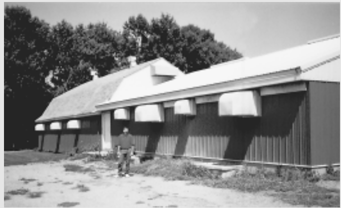
◆ Larry's barn remodeled for confinement operation.
