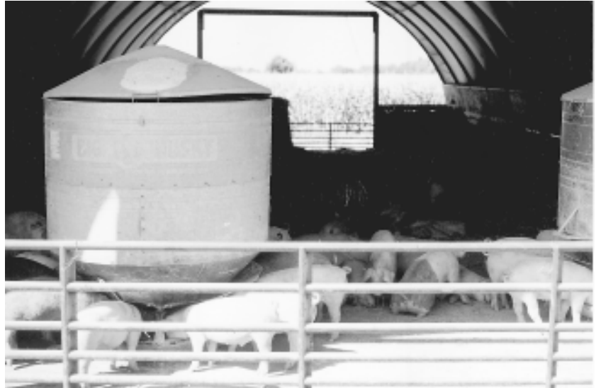
◆ A 30' x 72' hoop structure can accommodate more than 180 hogs.
