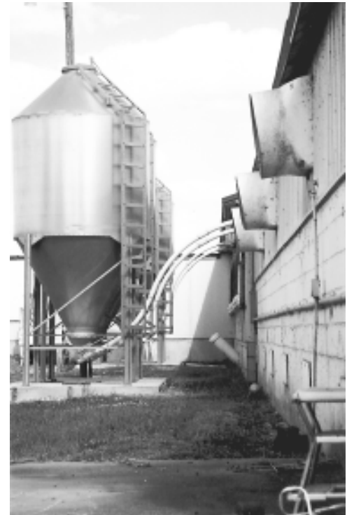
◆ Bulk feeder tanks are mounted to the outside of confinement facilities.
