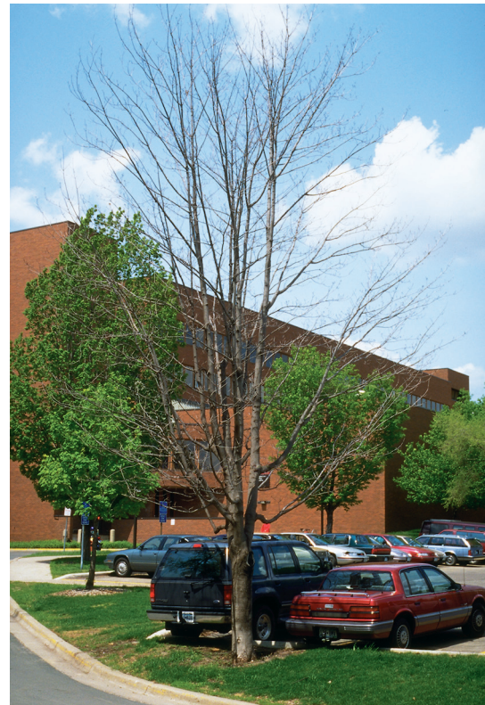
Fig. 12—Left, above: In 1994, this sugar maple exhibited significant stunt and dieback following a normal winter. There were 12 inches of soil over the main order roots and the stem circumference was significantly (> 50%) compressed by SGRs.
