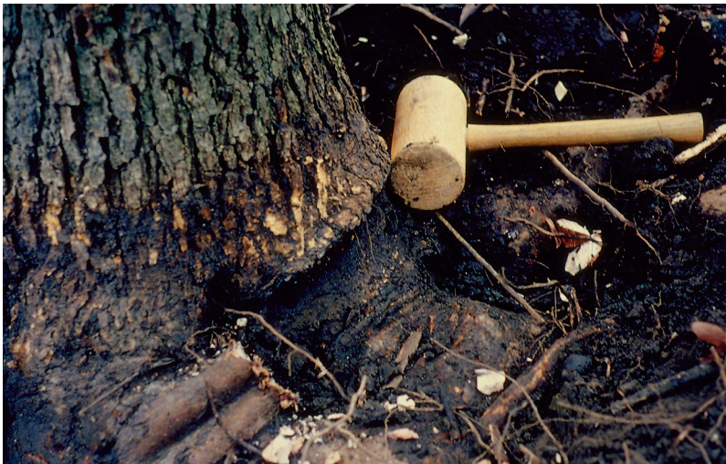
Fig. 35—Both SGRs were removed with a mallet and wood chisel. The excavated area was then lightly (2+ inches) mulched.
