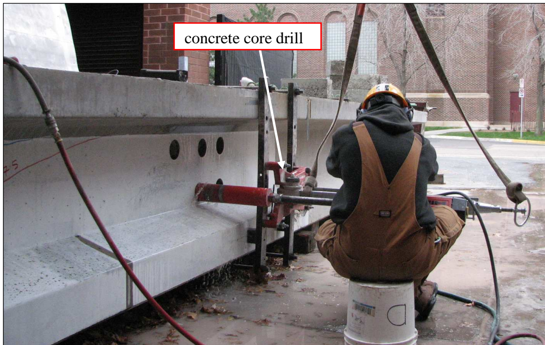
Figure D-6 Setup for taking concrete cores
