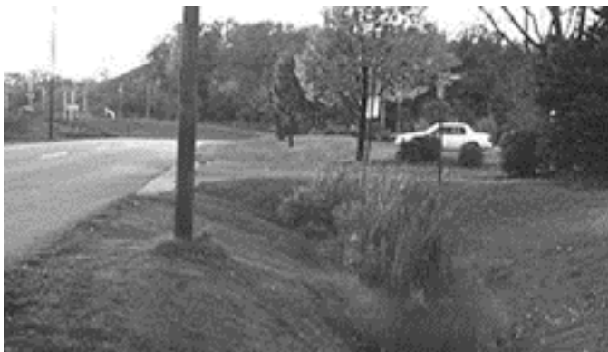
Figure 2.6b Picture and Schematic of a Wet Swale
