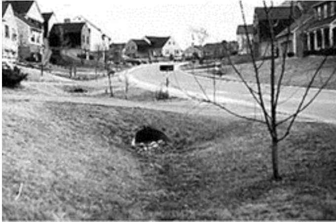
Figure 2.6a Picture and Schematic of a Dry Swale
