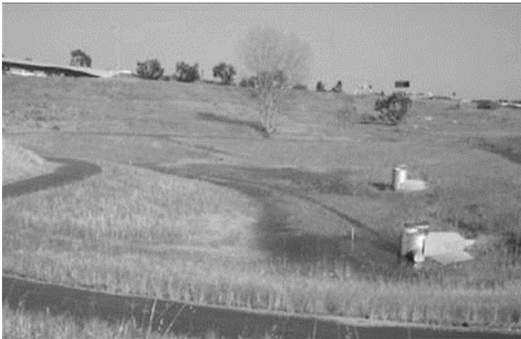
Figure 2.3 Picture of a Dry Pond
