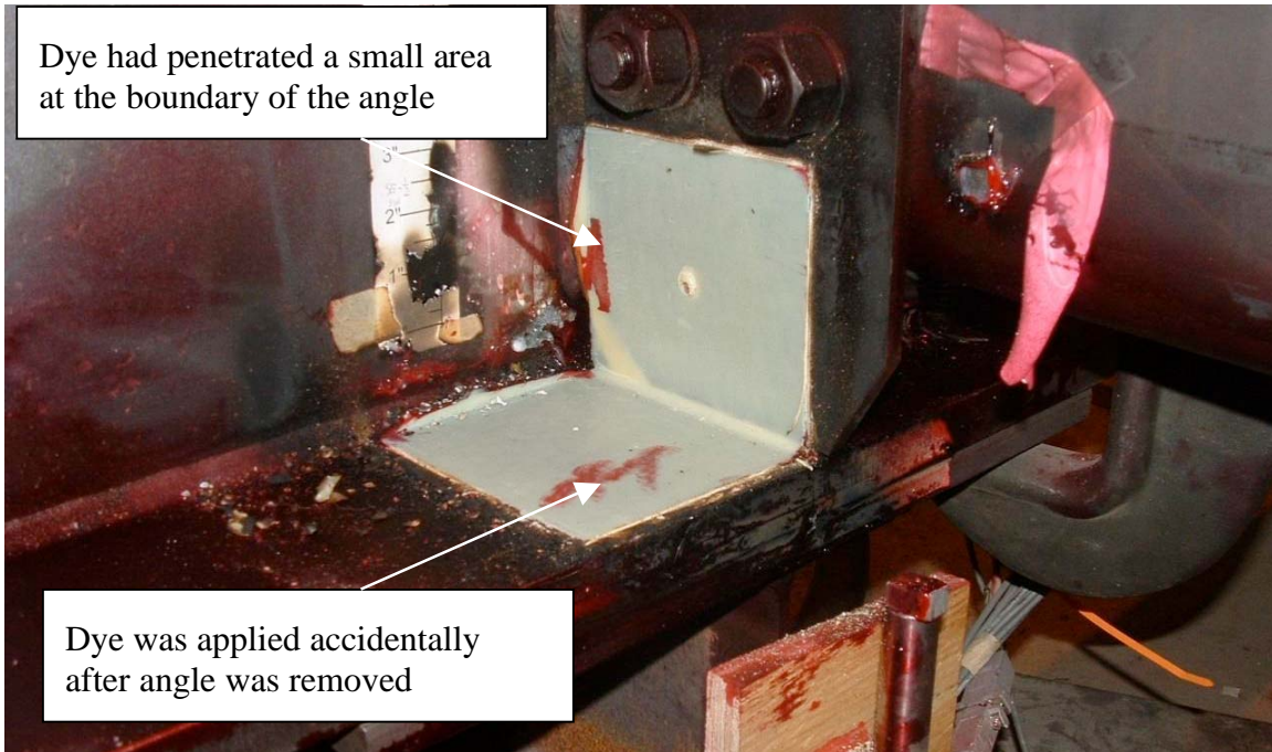
Figure 4.52 Detached angle at web gap SE-1/2
