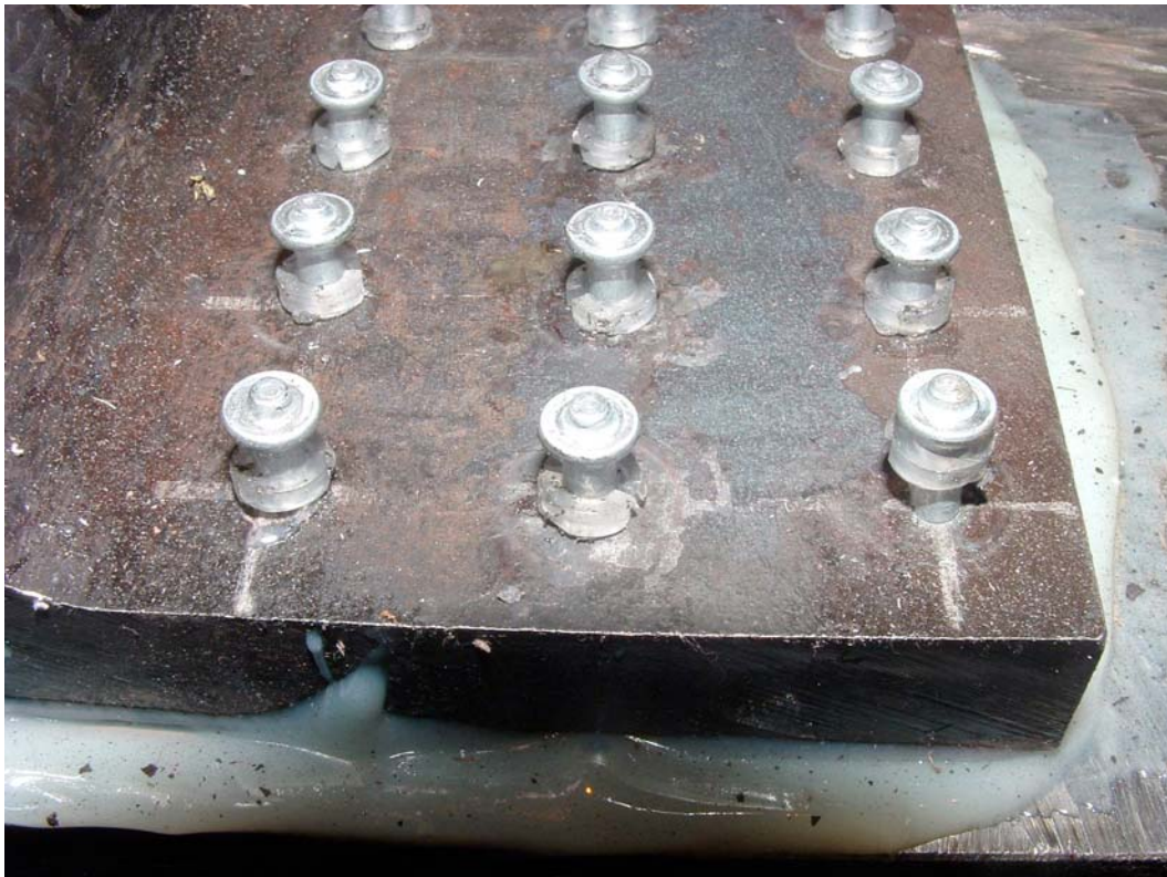
Figure I.2 Picture of the retrofit angle with Hilti powder actuated fasteners
