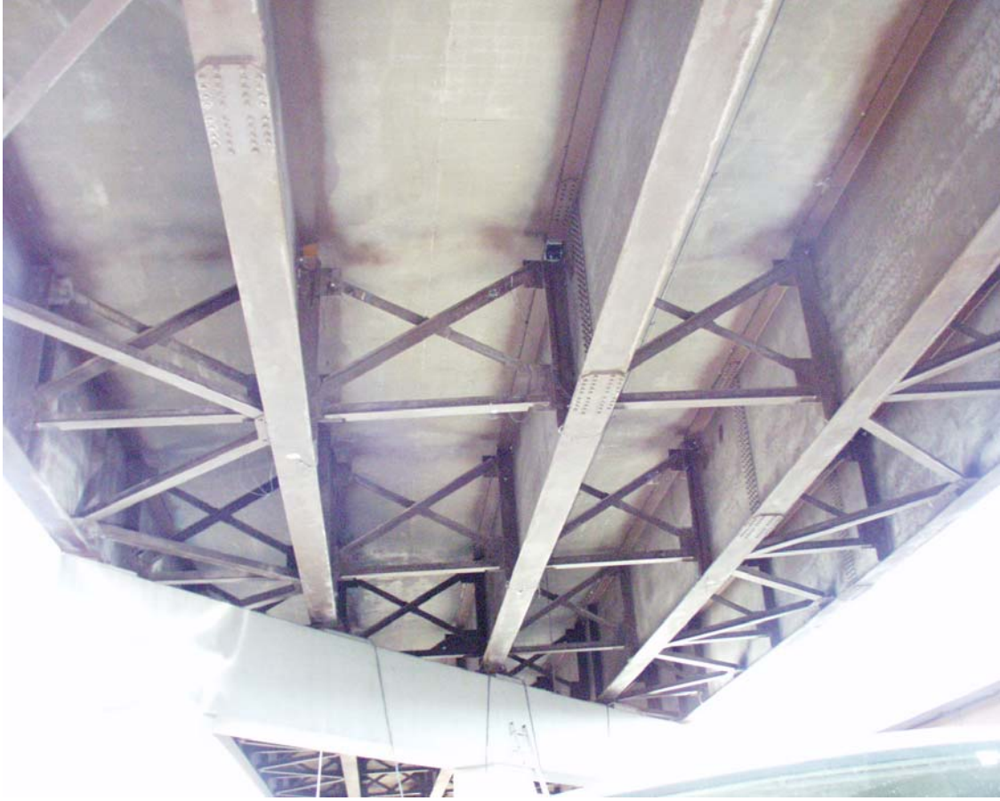
(c) Underside view of the CFD bridge (Bridge #27984)
