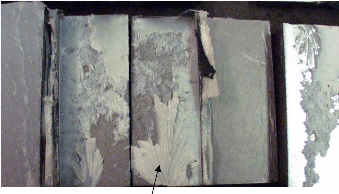
Adhesive became very brittle and formed cracks
