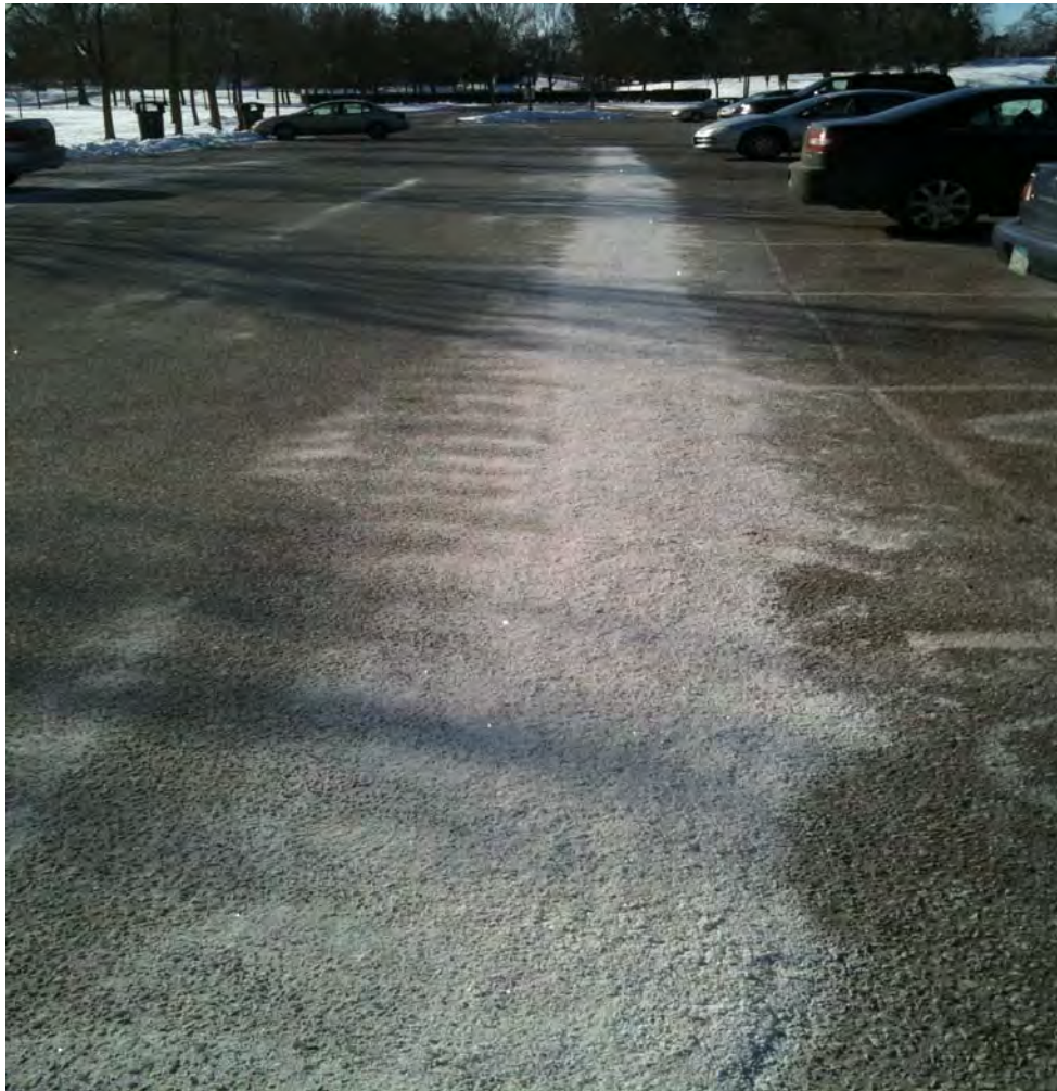
Photo 1: Excessive application of de-icing chemicals, Pavilion parking lot.
