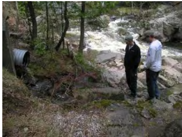
Figure 5: Storm drain entering Amity Creek.
