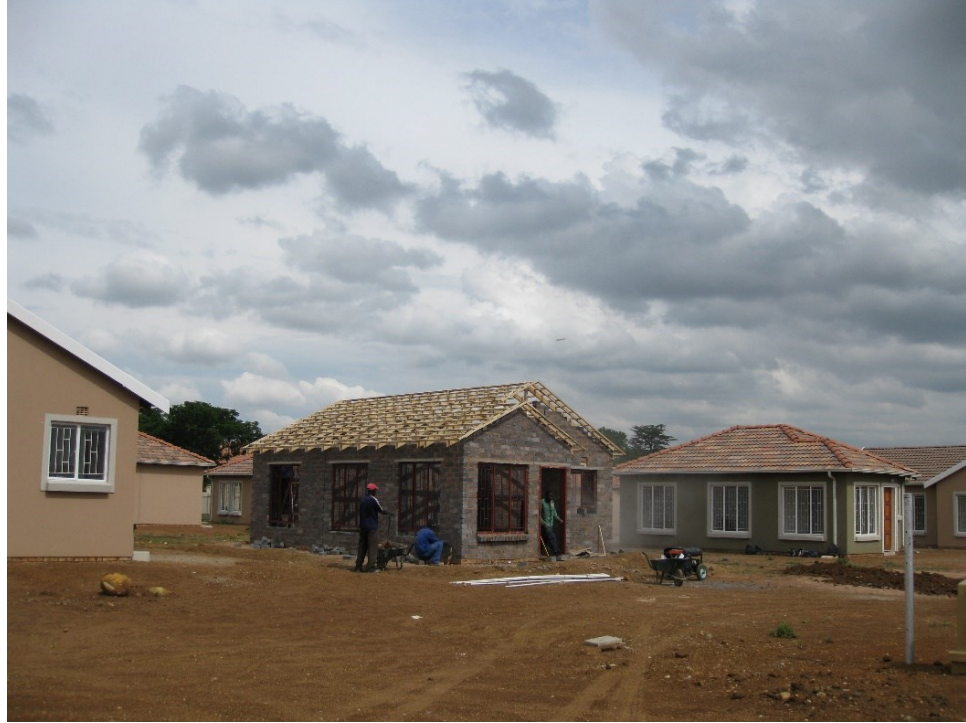
Figure 48: Phase 4 house in Alveda Park after roofing trusses laid (same house as Fig. 47)
