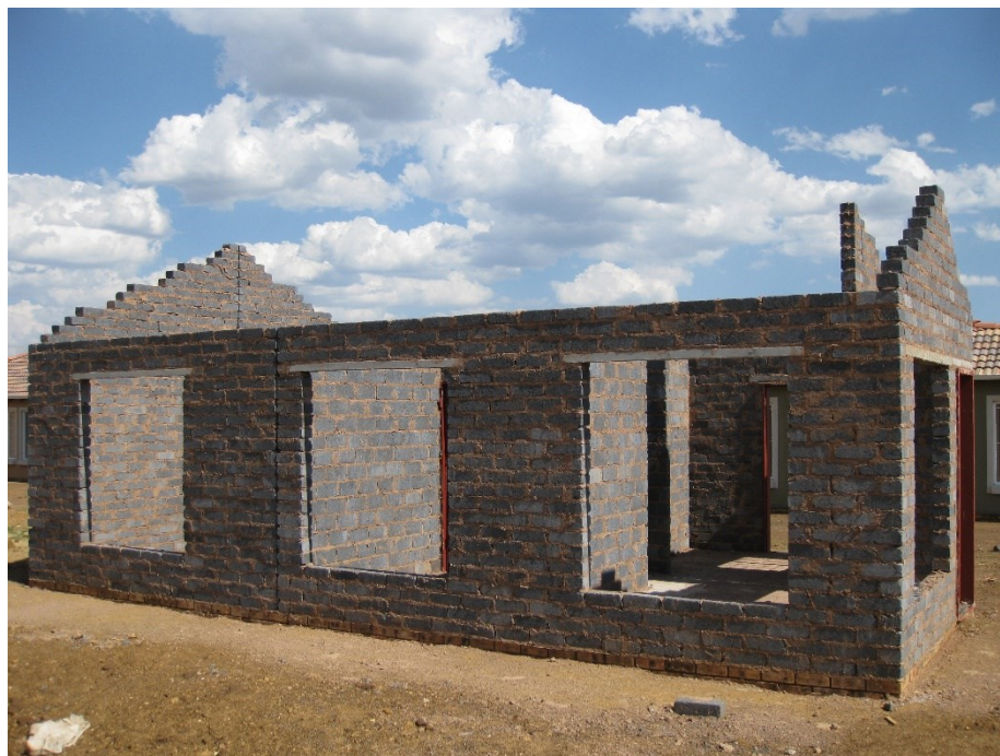
Figure 47: Phase 4 house in Alveda Park reaches roof height
