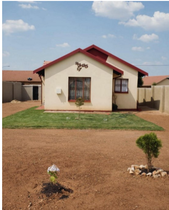
Figure 38: Protea Glen house, photo by Jodi Bieber (Bieber and Mhlongo 2010, 152)
