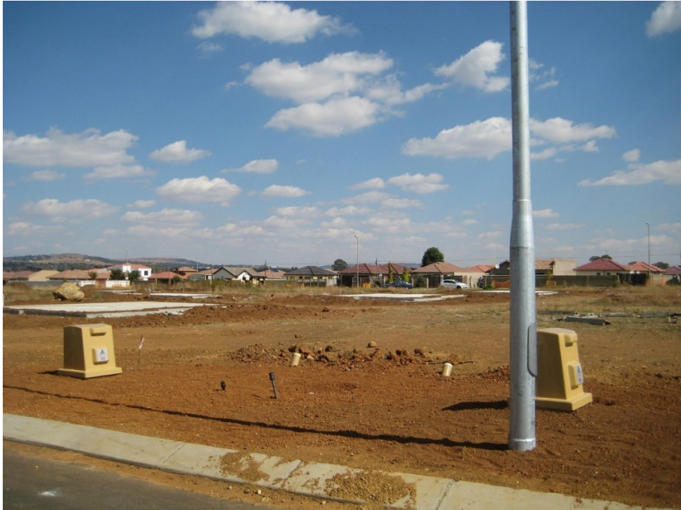
Figure 43: breaking ground on Alveda Park Phase 4; long-completed Phase 2 in the background. May 2013
