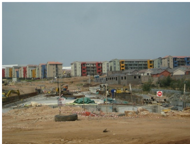
Figure 52: Fleurhof Integrated Human Settlement from the west bank, October 2012
