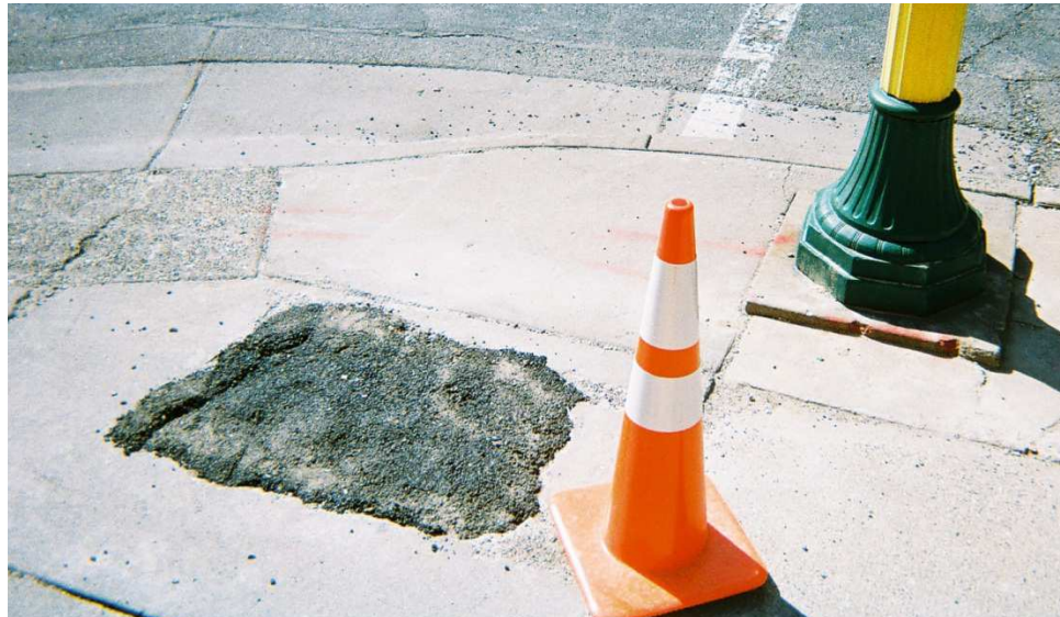
Figure 17: Sidewalk repair outside building
