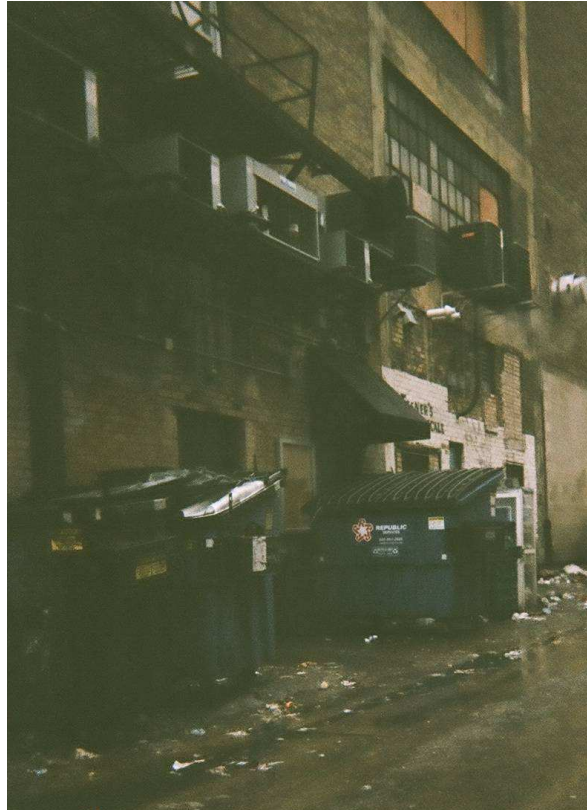
Figure 4: Picture of Alley behind building
