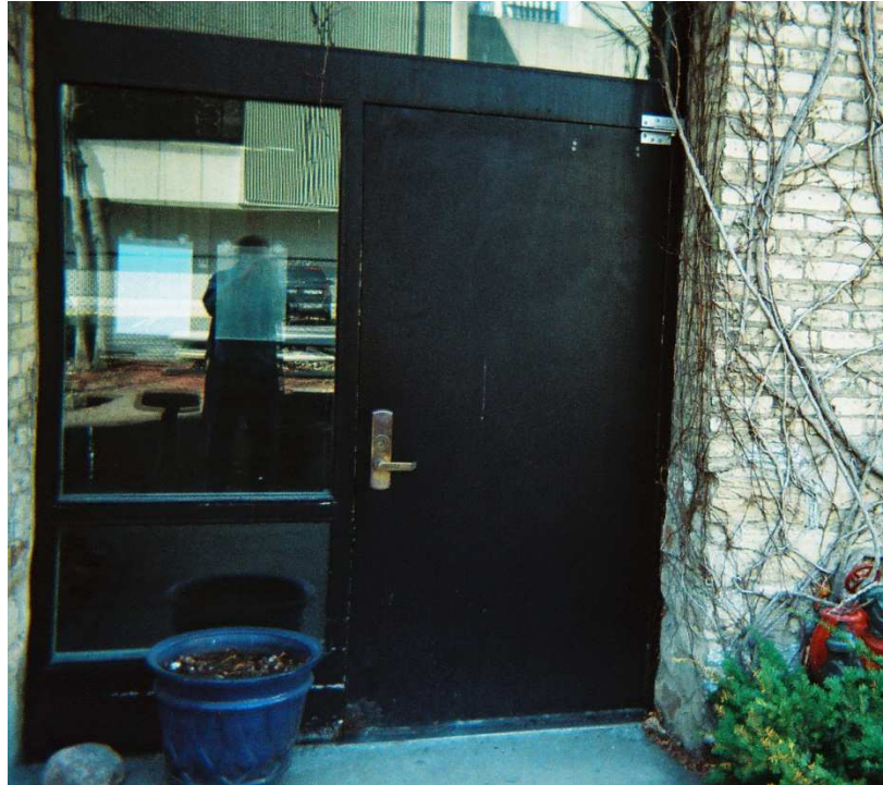
Figure 15: Door from courtyard -staff accessible
