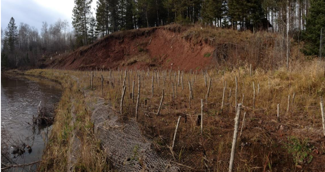
Figure 3.2: Toe Wood Structure at BHHR in November 2015.
