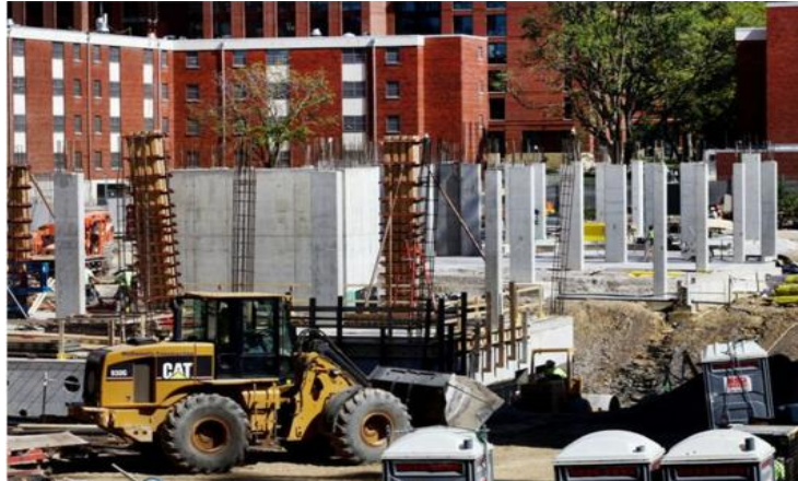
Figure 36. “Dormitory Construction in Columbus.” North Dorms in the background, new dorms under construction in the foreground. Source: Image by Fred Squillante, Columbus Dispatch , in Mary Morgan Edwards, “Ohio State’s new dorms offer spaces for community experiences,” Columbus Dispatch , September 28, 2015. 420
