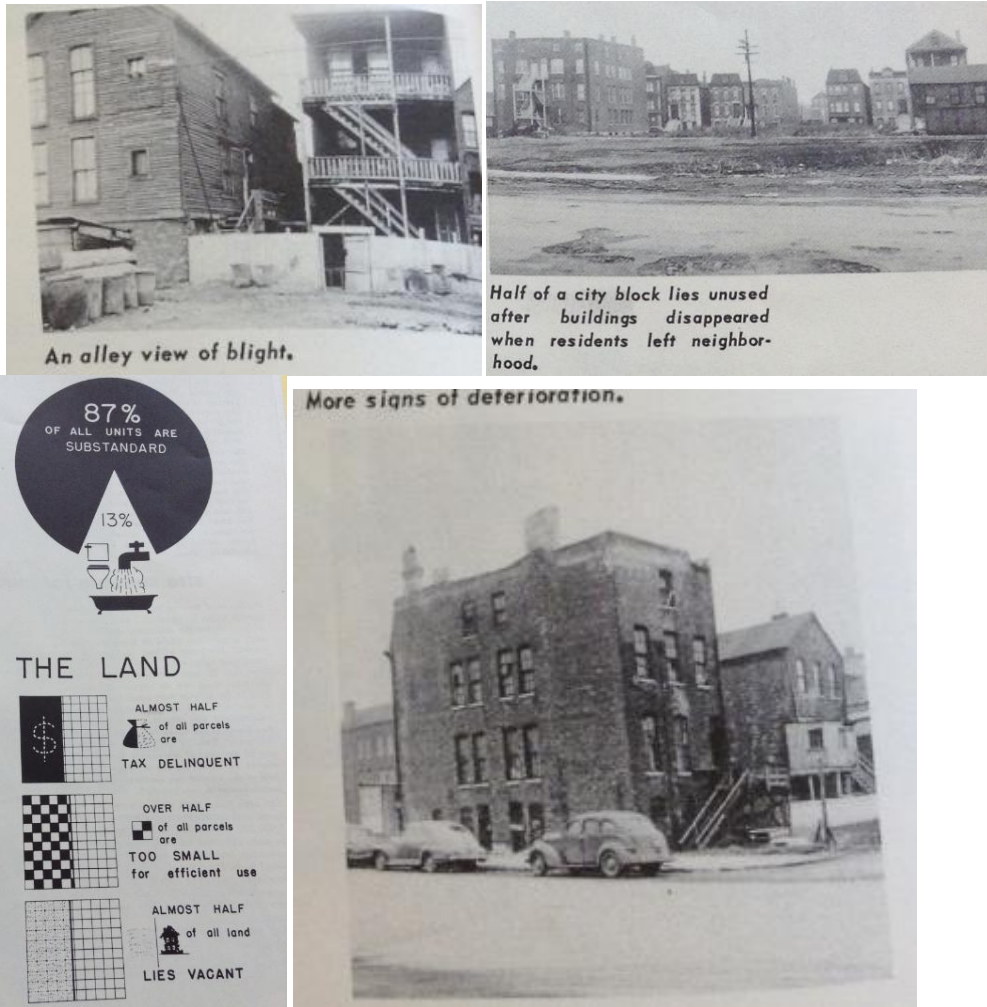
Figures 27-30: Illustrations of Blight on the Near West Side. Source: Chicago Land Clearance Commission, Redevelopment Project Number Three , June 1951, in Folder: "Redevelopment Projects-Project # 3- West Side Industrial, 524-4414," Box 524-783, Series III: Planning and Urban Renewal, Metropolitan Planning Council Records, The University of Illinois at Chicago, Chicago, IL.
