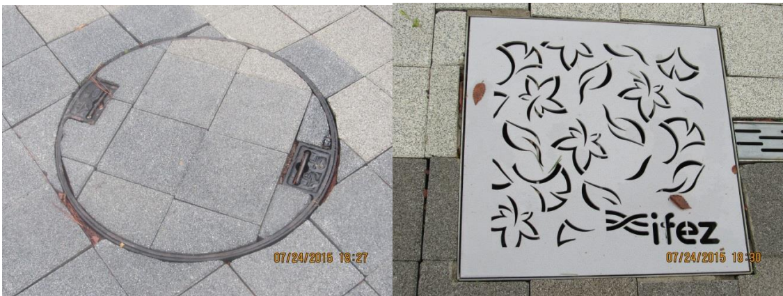
Figure 6: Two drainage covers in Central Park
