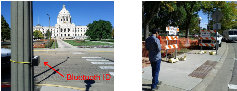
Figure 4-11 Installation of Bluetooth Beacon at Field Test Site (N. Sidewalk)
