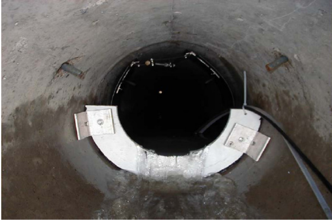
Figure 5: Circular weir installed in outlet pipe of Pond.
