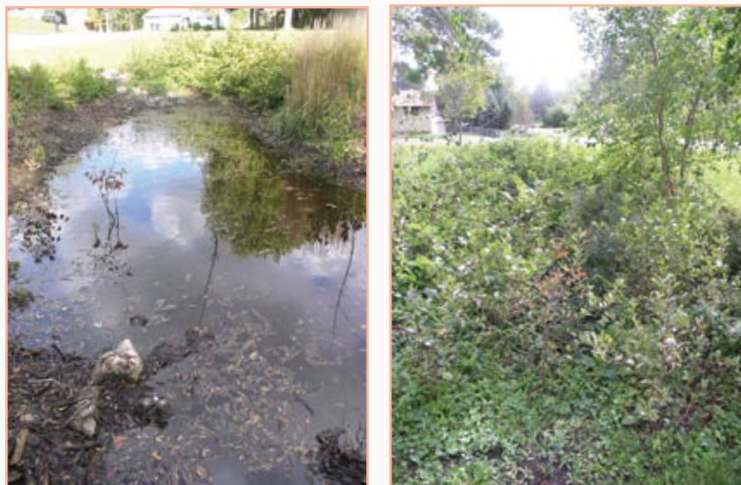
Figure 3.1: Examples of visual inspection for a rain garden that is not functional (left) and a rain garden that is functional (right).
