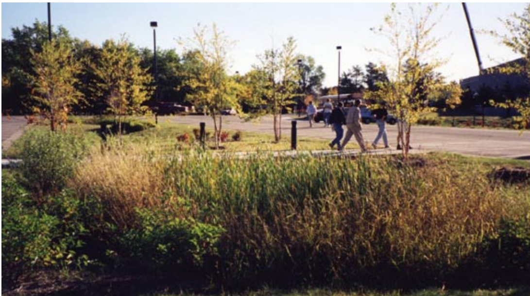
Figure 1: Vegetated infiltration median strips.
