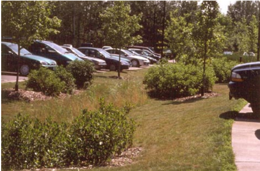
Figure 3: A wetland system that provides depression storage, infiltration, and vegetative filtration.
