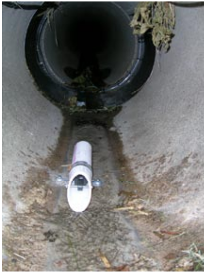
Figure 1: Installation of a temperature probe in a sewer pipe.
