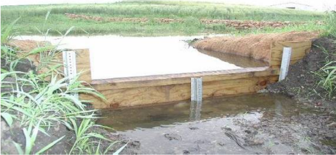
Figure 4: Rectangular weir at inlet of Pond #3.
