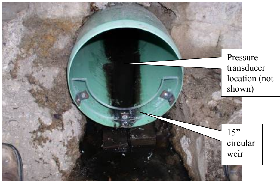
Figure 3: Pre-calibrated 15-inch circular weir installed downstream of the V2B1. Pressure transducer and transducer anchoring not shown. This weir location provided free outfall conditions at all flow rates due to the PVC pipe's favorable elevation vs. the existing 36-inch RCP it discharged into.
