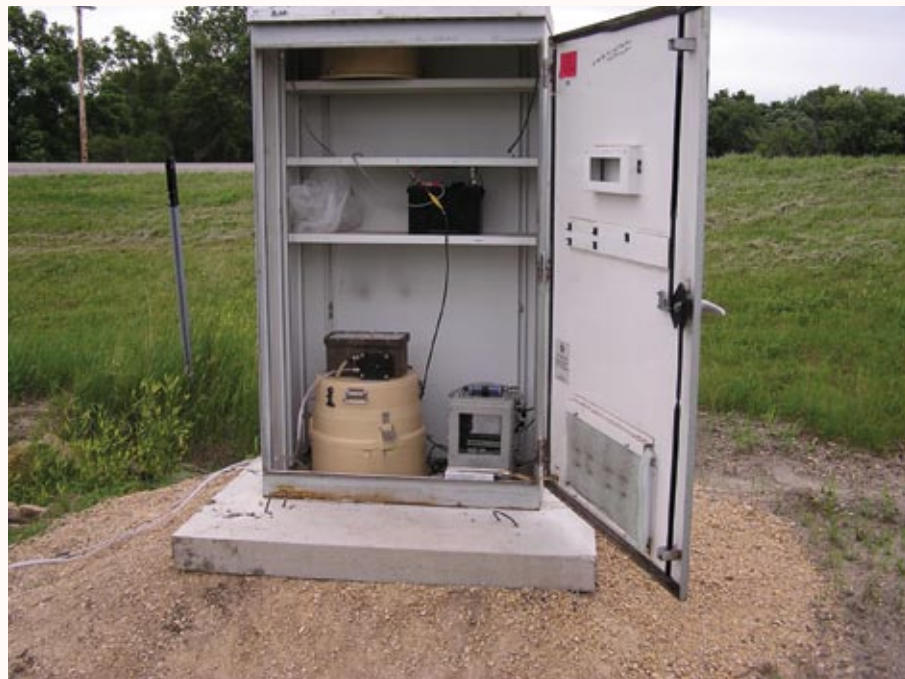
Figure 5.8: Protective cabinet housing automatic sampling equipment.
