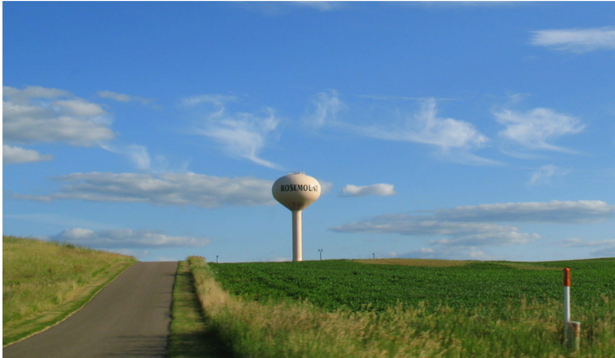
FIGURE 1: ROSEMOUNT WATER TOWER AS PHOTOGRAPHED BY THE TWIN CITIES DAILY (2008)
