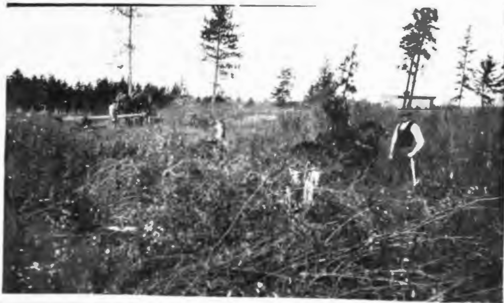
Fig. 12 Pulling stumps by stump puller method.
