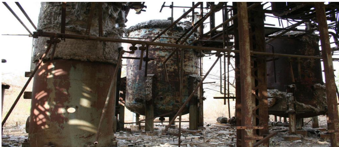
Figure 1.2: Deteriorating section of the MIC plant, decades after the gas leak (By Simone.lippi at it.wikipedia [CC BY-SA 2.0 ( http://creativecommons.org/licenses/by-sa/2.0 )], from Wikimedia Commons) [25]
