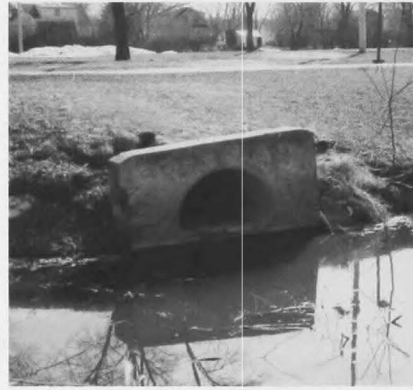
Stormwater culvert & headwall.
