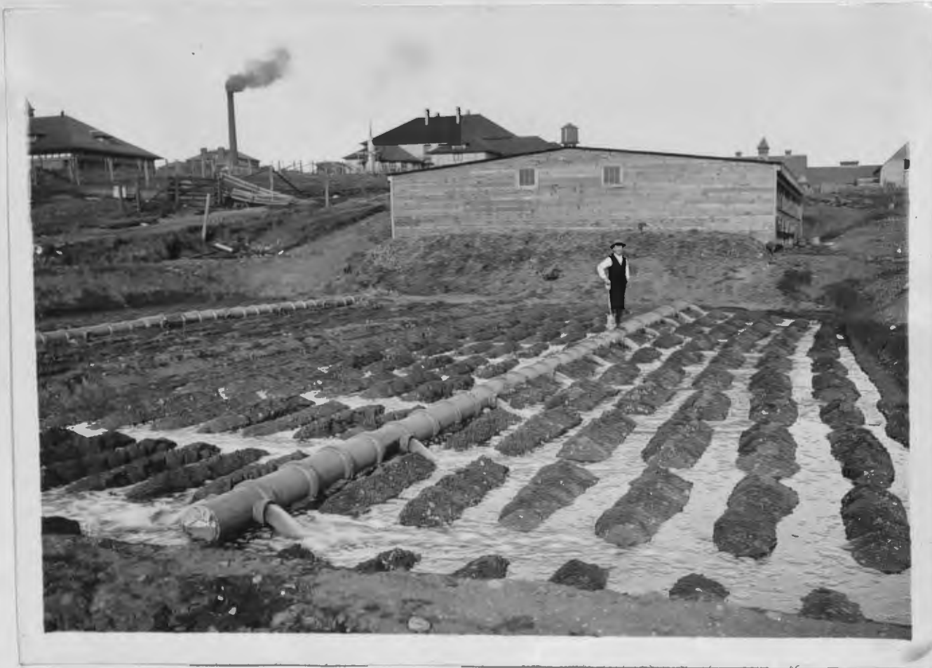
SAND FILTER BEING DOSED WHILE FURROWED FOR THE WINTER ALSO SIDE DOOR ON PERCOLATING FILTER OPEN
