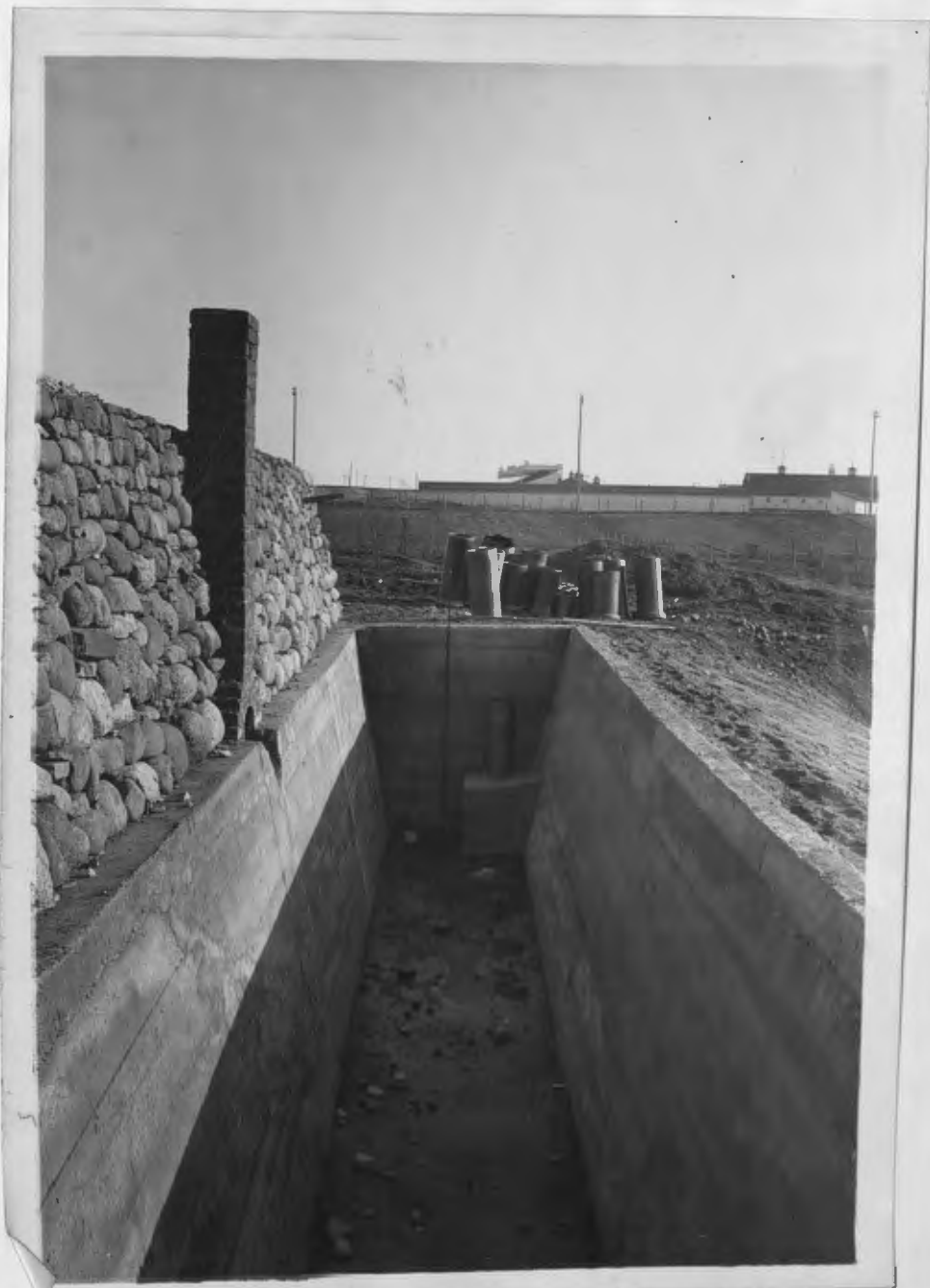
SETTLING BASIN PERCOLATING FILTER BEFORE BELL WAS PLACED ON SIPHON
