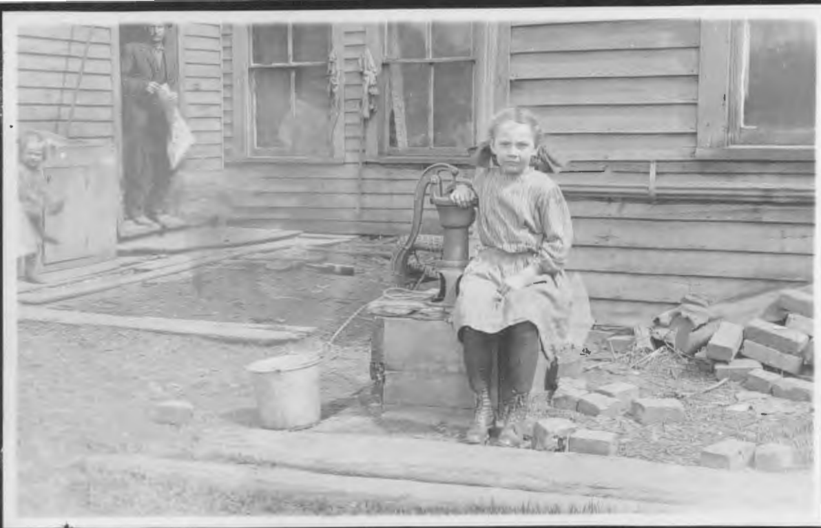
Thirty-one - a cistern water supply for three families. (rotten and full).
