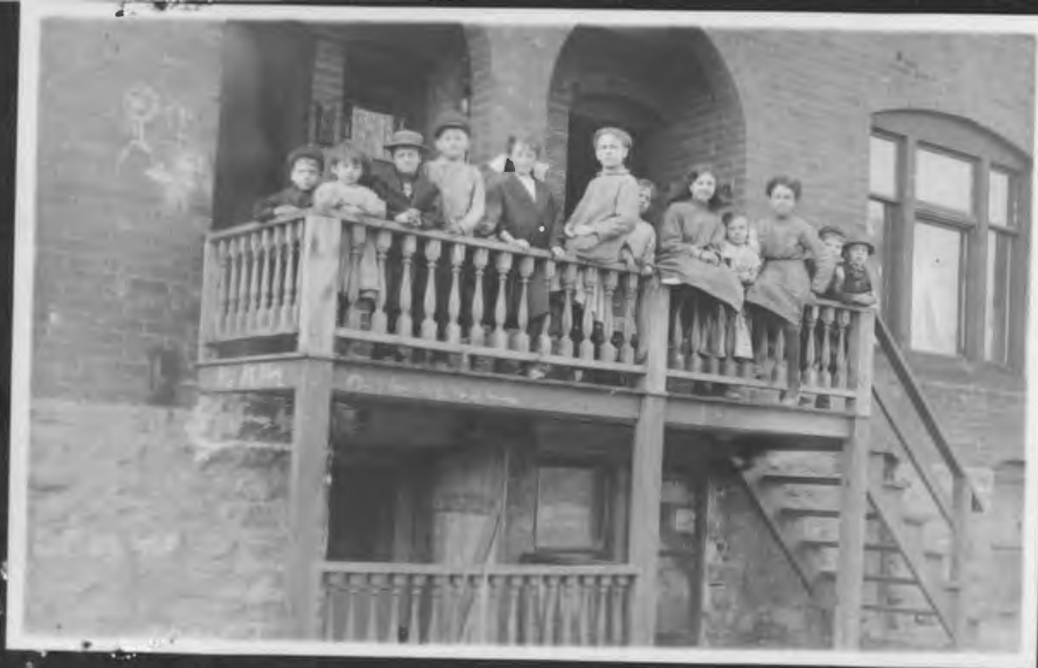
Nine - Children - and dark rooms Basements,
