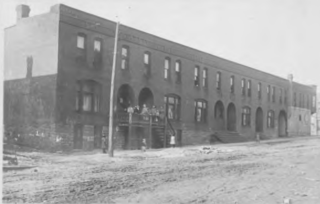
A tenement with dark rooms and basement apartment.
