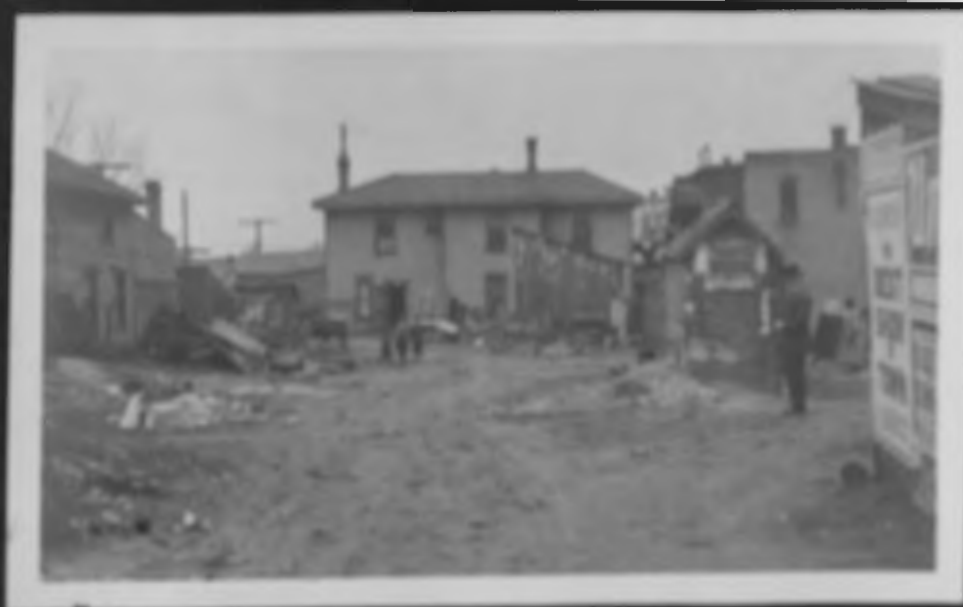
Forty-three. Dilapidated negro quarters.
