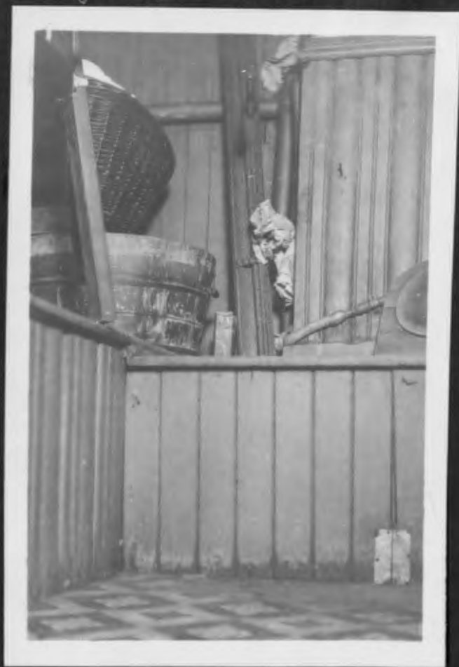
Twenty-eight - Dark closet and rotten enclosed plumbing.
