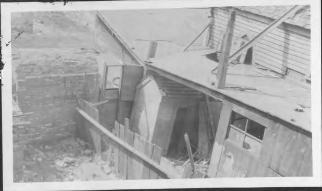
Twenty-nine - neglected and now ruined vault.
