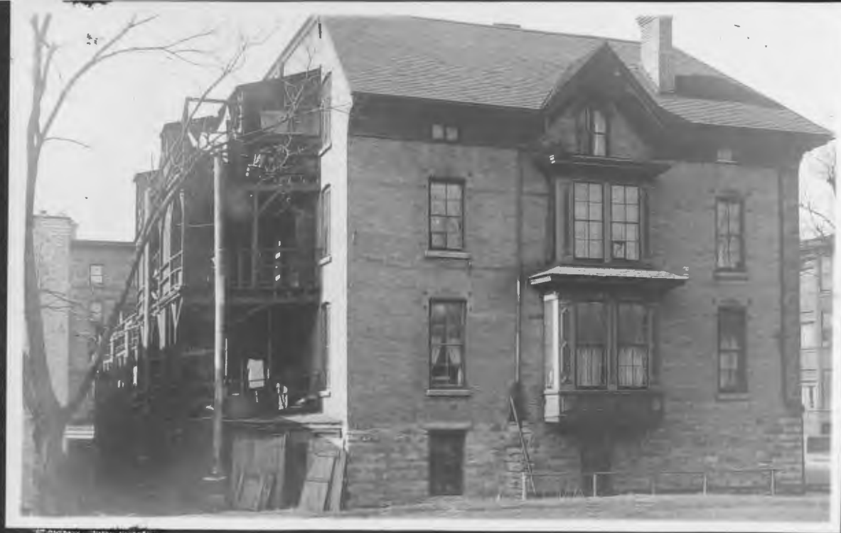
Eleven - Mark rooms basements,
