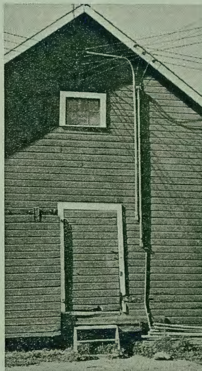
Service Entrance Switch in Granary
