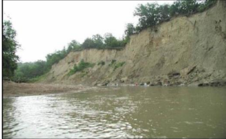
Figure 2. A steep tall bank actively sloughing along the Le Sueur River in Blue Earth County, Minnesota. Accumulated material at the toe is from past bank sloughing from above. Lack of vegetation on part of the bank indicates active sloughing nature of this bank.
