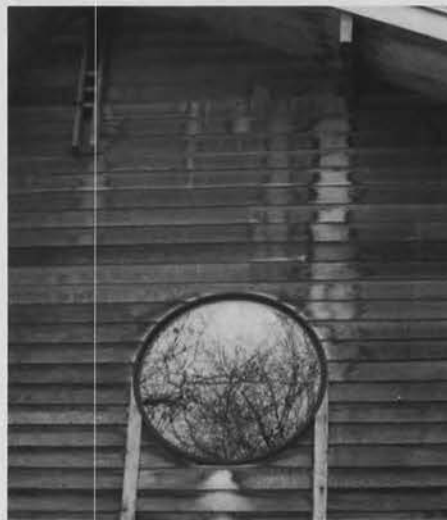
Figure 1. An exterior photo of a home with cathedral ceilings and bad moisture staining of siding due to an inadequate air barrier.
