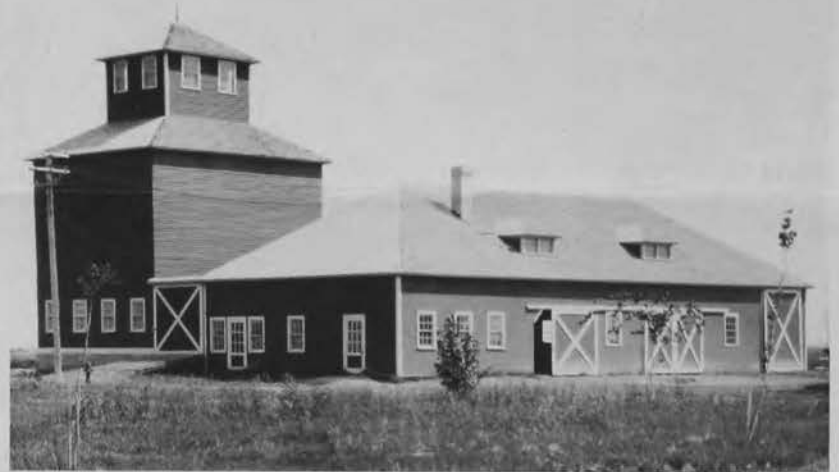
Machine shed and elevator were built the same year, 1913. Both buildings have since been replaced.
