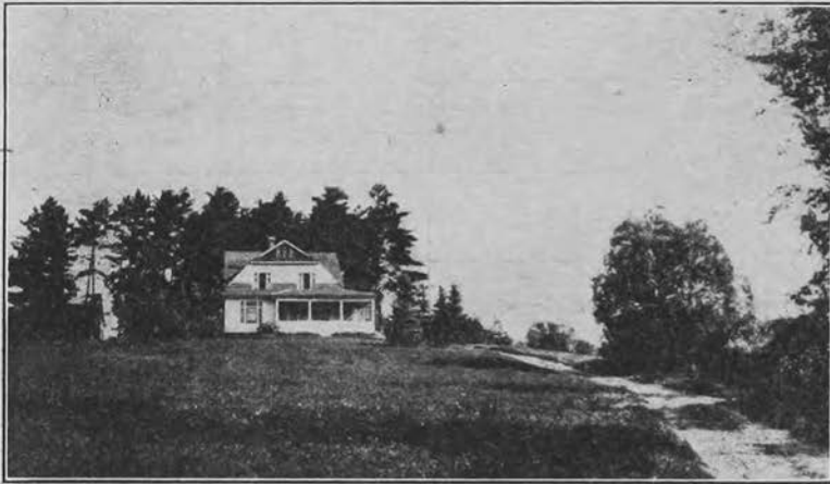
Fig. 2. Superintendent's Cottage From Entrance to Station
