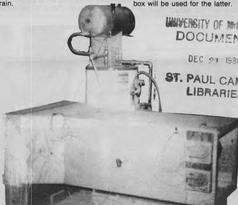
Experimental inlet air tempering system serving one room of station farrowing facility.
