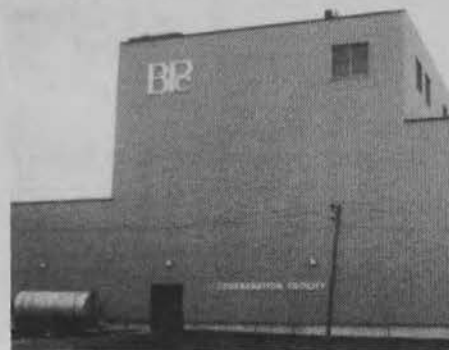
Blandin CoGeneration plant supplies ash for area farms.
