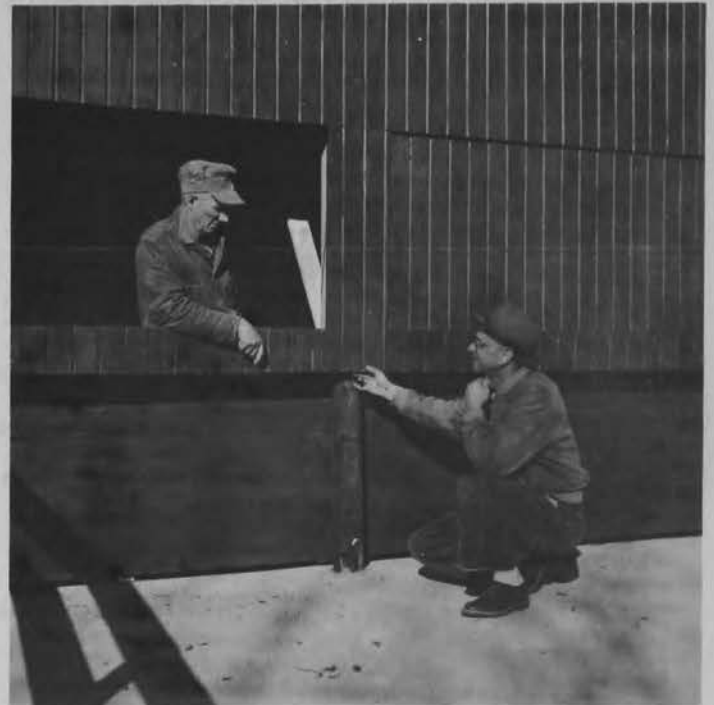
Harvey Holst, left, and Don Hasbargen, Mower county agent, inspect the construction in Holst's new pole-type hog house.
