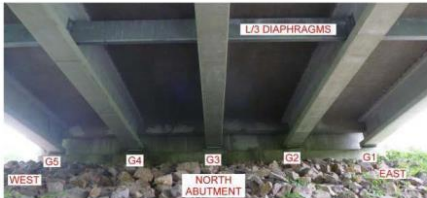
Figure 8. North Abutment Girder Numbering
