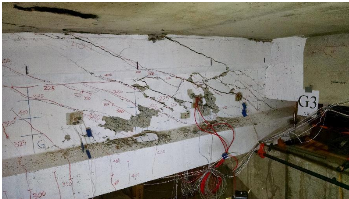
Figure 5-14. Web-Shear Crushing and Deck Punching in G3 during LBUW Looking South
