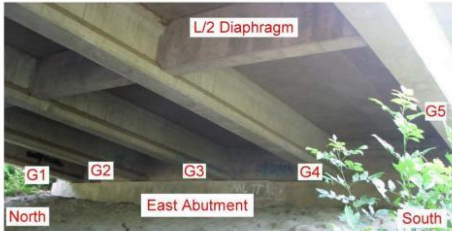
Figure 8. East Abutment Girder Numbering
