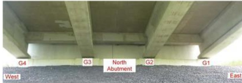
Figure 10. North Abutment Girder Numbering
