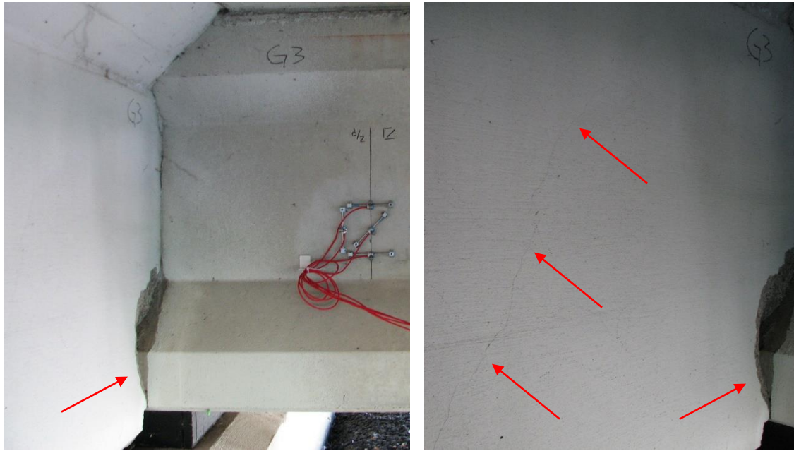
Figure 5-12. End Diaphragm Cracking Observed in Field Bridge 73872
