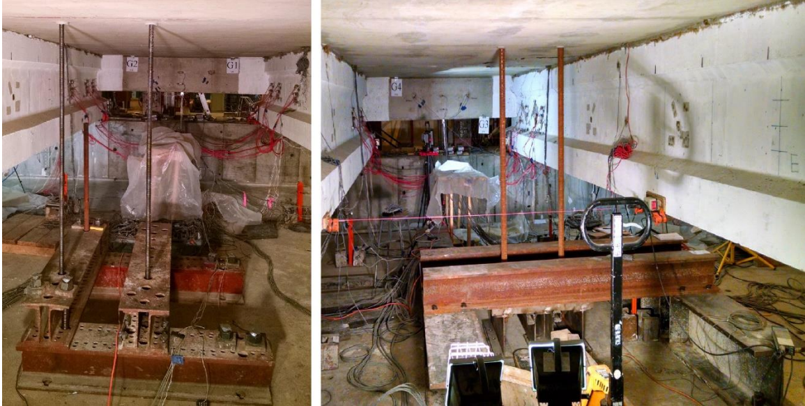
Figure 4-35. Load Frame Tie-Down Systems at Midspan below Bridge Deck Looking West during LBUW
