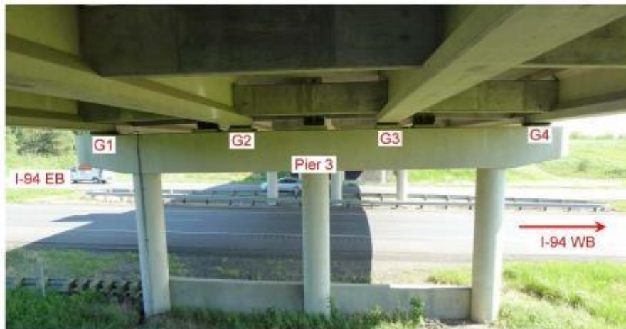
Figure 11. Pier 3 Girder Numbering
