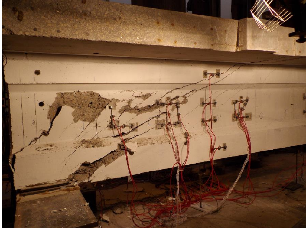
Figure A-14. Web-Shear Crushing Failure in 30.75 ft Span
