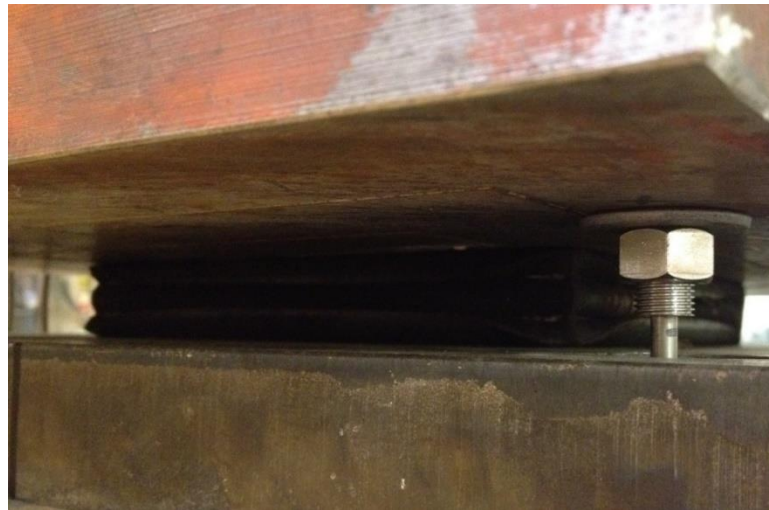
Figure E-11. Bulging Observed in 1-3/8 in. Bearing Pad
