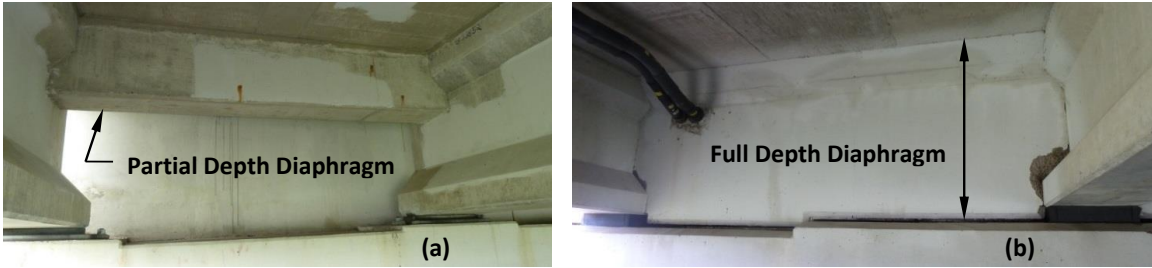
Figure 6-1. (a) Partial Depth and (b) Full Depth Diaphragm with Interface Cracking
