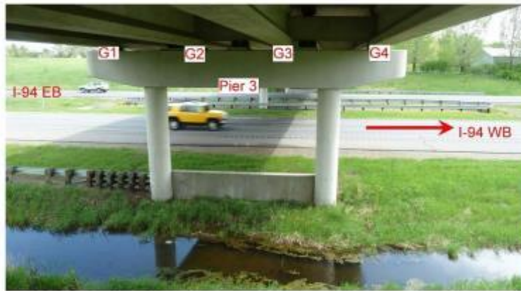
Figure 11. Pier 3 Girder Numbering
