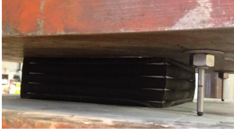
Figure E-14. Bulging Observed in 2-1/2 in. Bearing Pad
