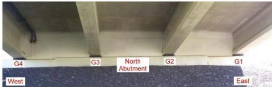
Figure 10. North Abutment Girder Numbering
