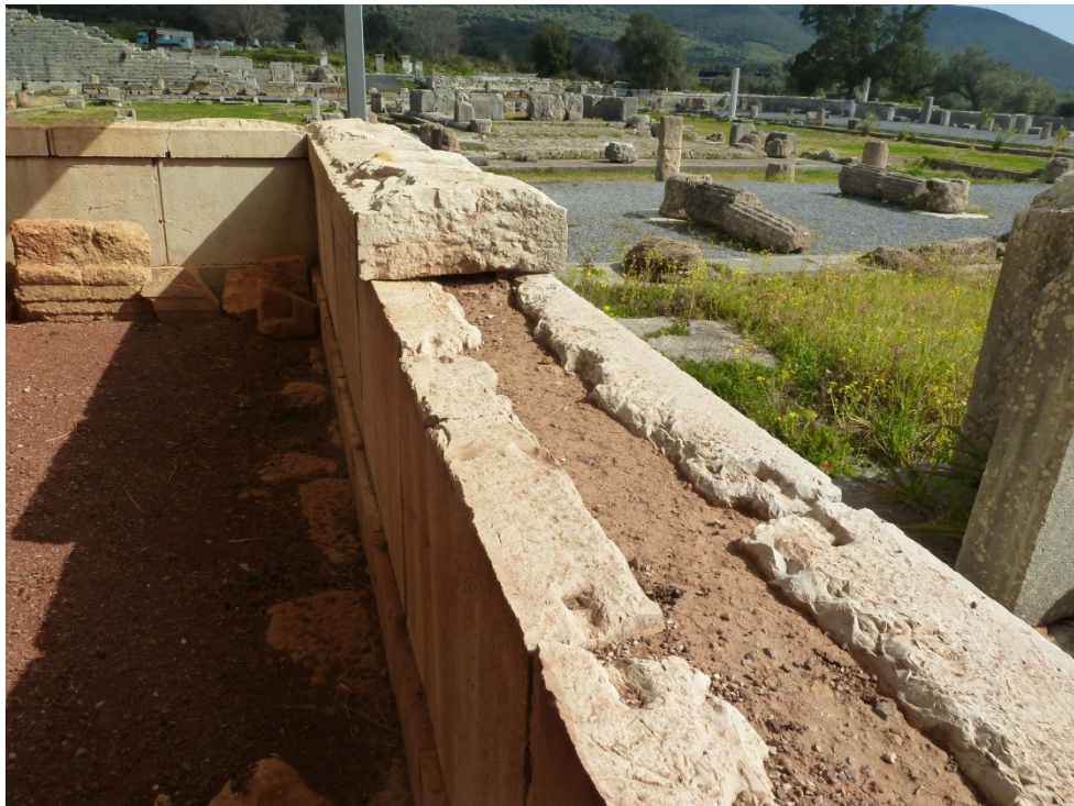
Fig. 66 Messene – double curtain orthostate wall with orthostate crown
