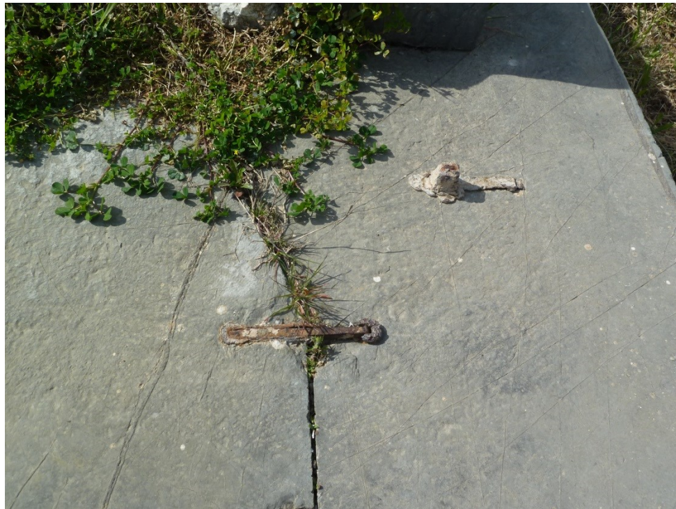
Fig. 62 Messene – clamp and dowel still in place
