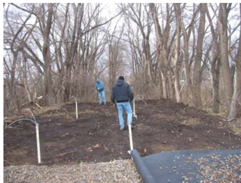
Figure 3. Bark bed installation.
