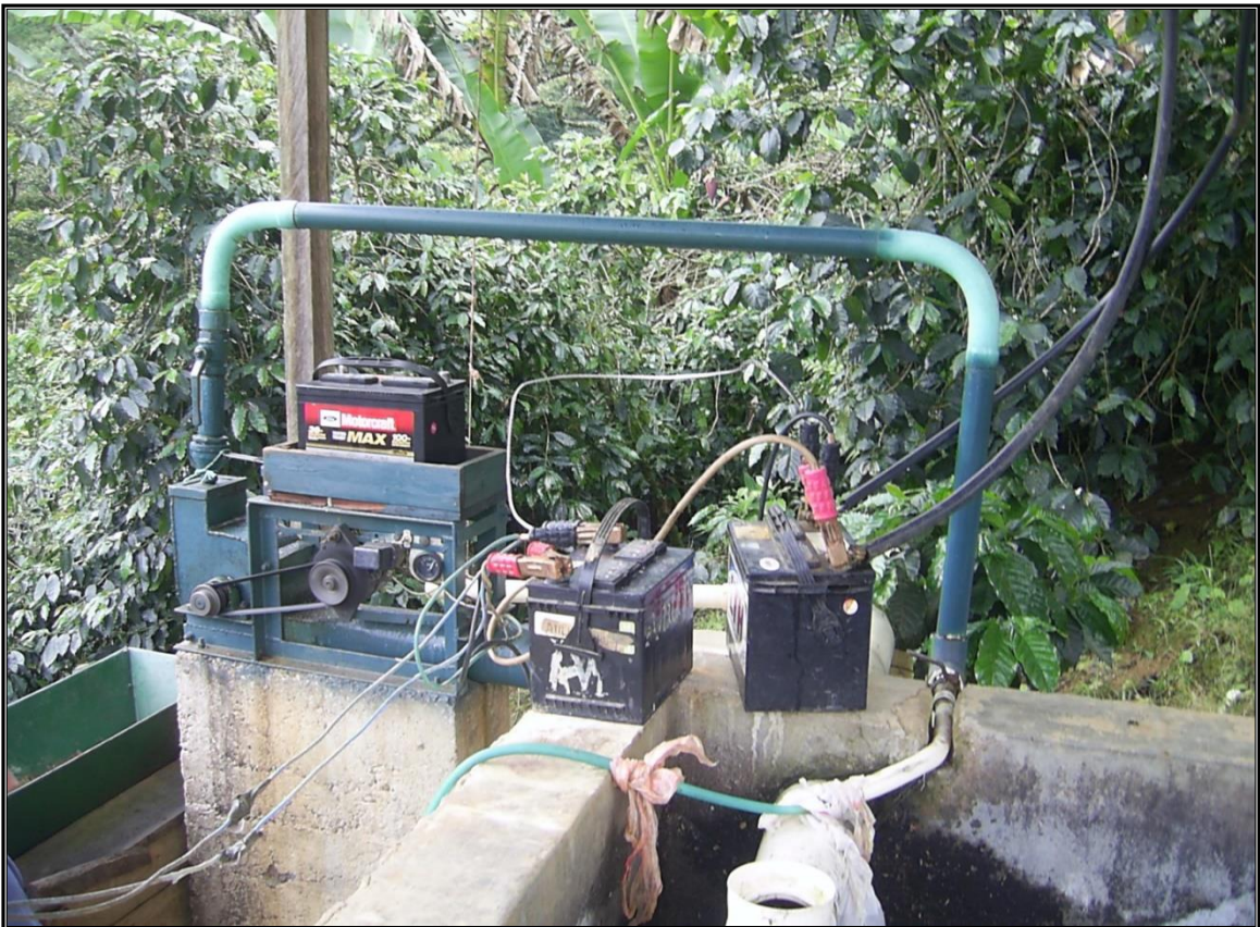
Figure 4.10: Using a Microturbine to Charge Automobile Batteries Source: Jeff DeGrave, 2012
