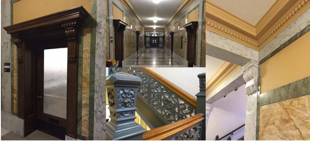
Figure 7. Folwell Hall restored main floor corridor
