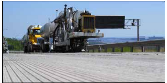
Next Generation Concrete Surface, also known as innovative diamond grinding, was used on I-35 in Duluth, Minnesota.
