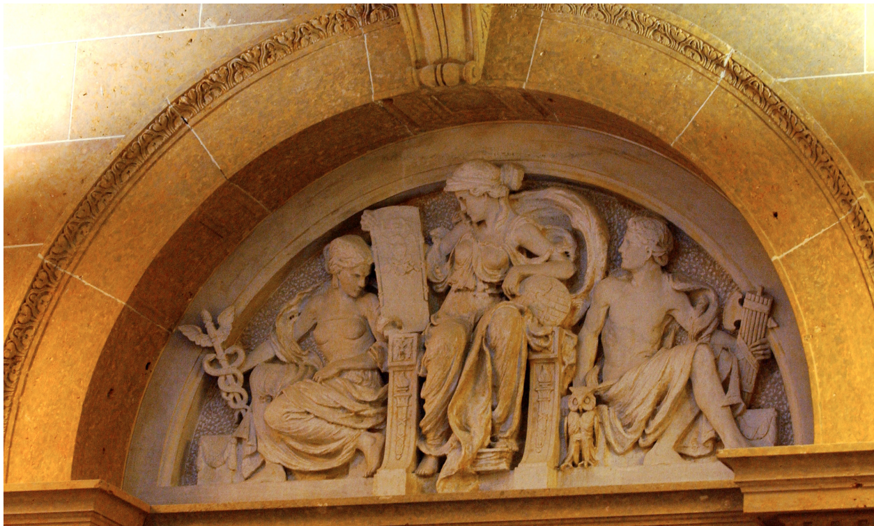
Architectural detail at Walter Library.
