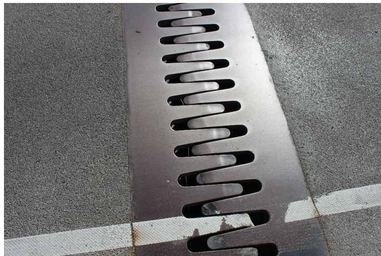
Figure 50: Expansion Joint on Bridge 9066
