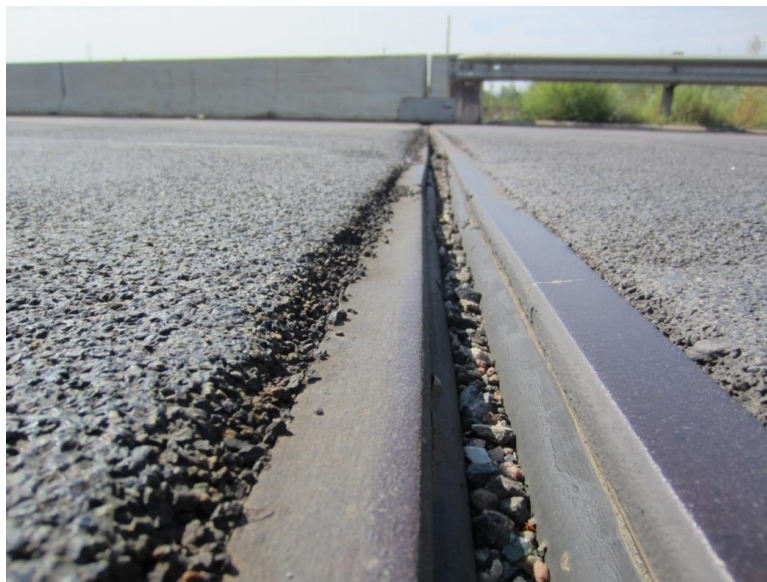
Figure 34: Joint Abrasion on Bridge 69006 (Traffic Moves from Left to Right)
