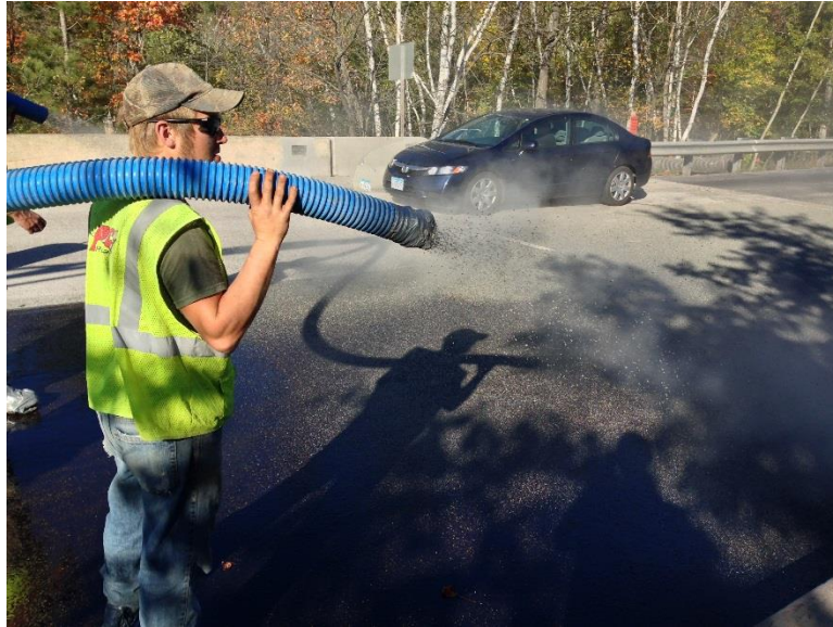
Figure 4: Aggregate is sprayed onto the Layer of Epoxy
