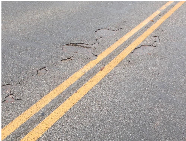
Figure 46: Delamination of Transpo System on Bridge 6347 along Centerline
