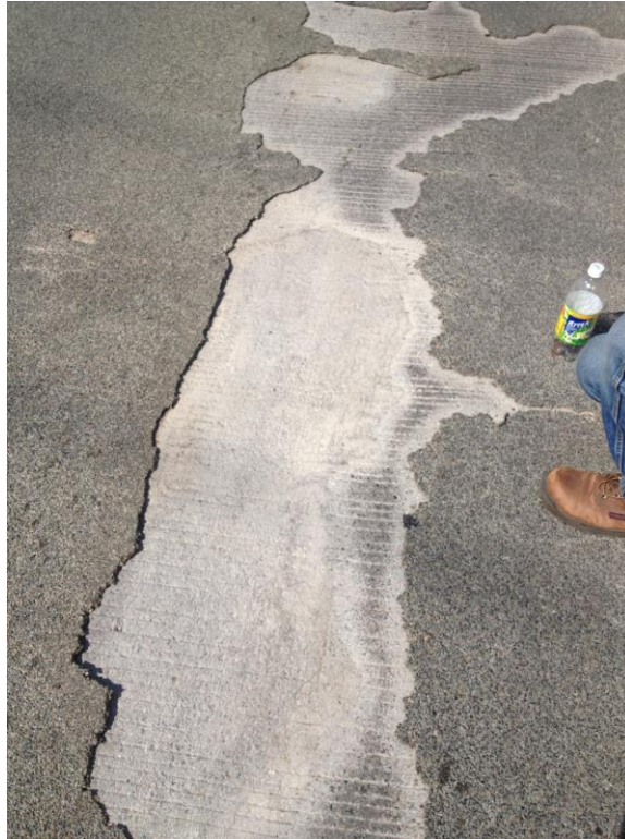
Figure 47: Delamination of HFO on Robert Street Bridge (Br 9036)
