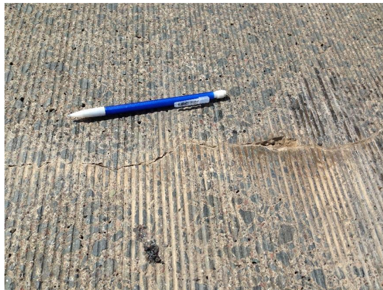
Figure 73: Area of Bridge 9824 Tested for Permeability
