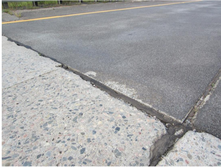
Figure 36: Damage near Approach Panels on Poly-Carb System (Bridge 69006)
