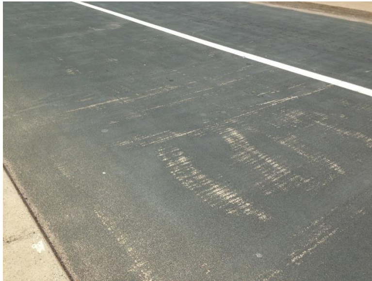
Figure 30: Excessive Snow Plow Abrasion (Br 27758)
