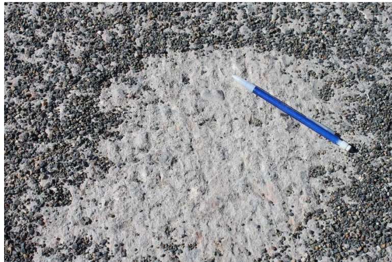
Figure 1: Sandblasting a Concrete Deck to Prepare the Surface for an HFO System
