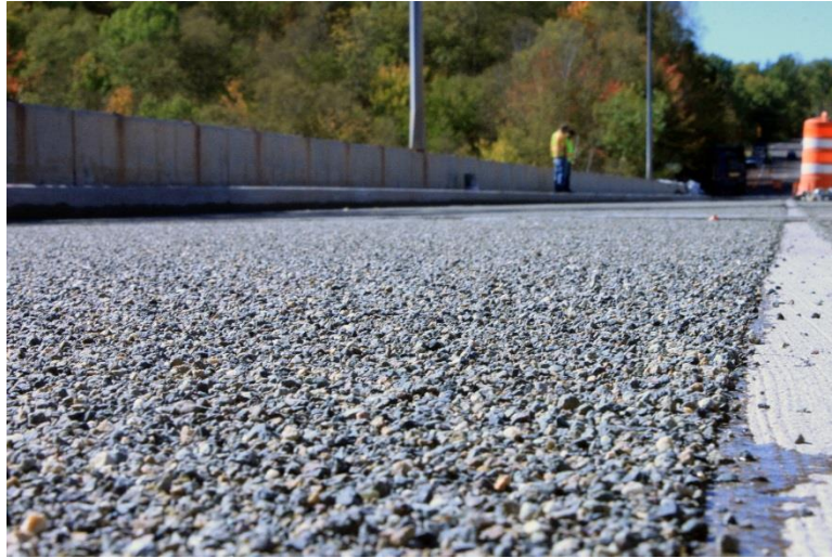
Figure 6: Final Epoxy HFO System (Left Side: Epoxy HFO Lane, Right Side: Concrete Deck that Still Requires the Placement of an HFO Surface)
