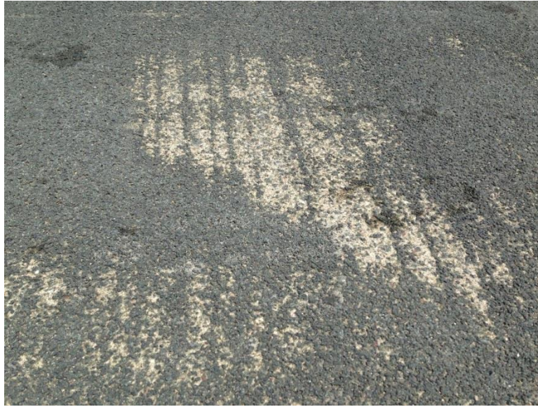
Figure 31: Thin Epoxy System (Br 27758)
