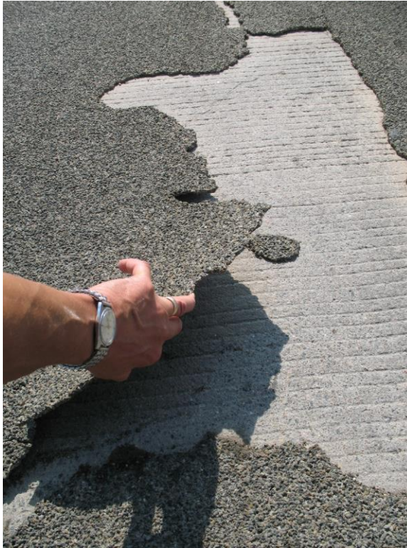
Figure 48: Minimal Bond Strength Existed in the Distressed Areas (Br 9036)
