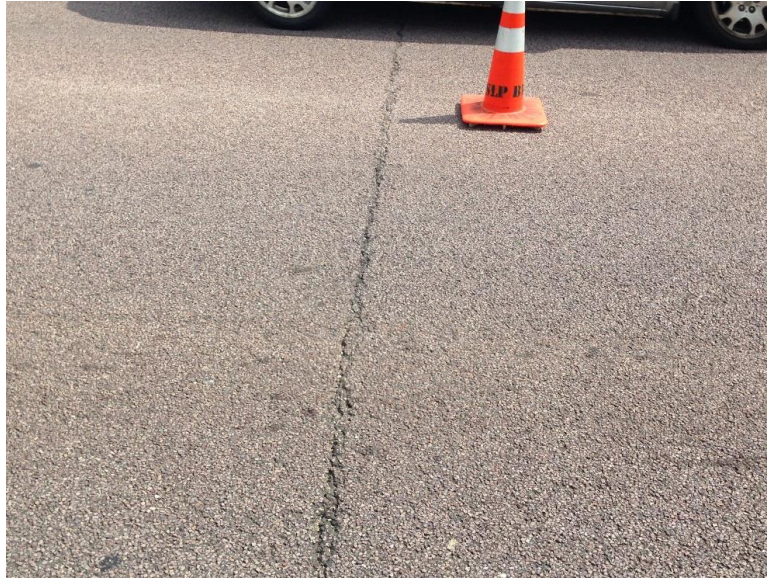
Figure 44: Longitudinal Crack in Novachip System (Br 27019)
