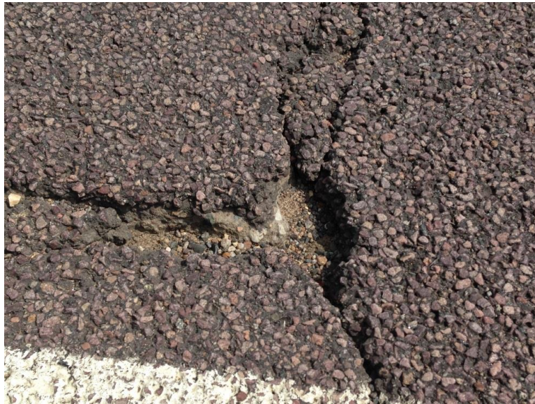
Figure 45: Reflective Cracking in Novachip System (Br 27019)
