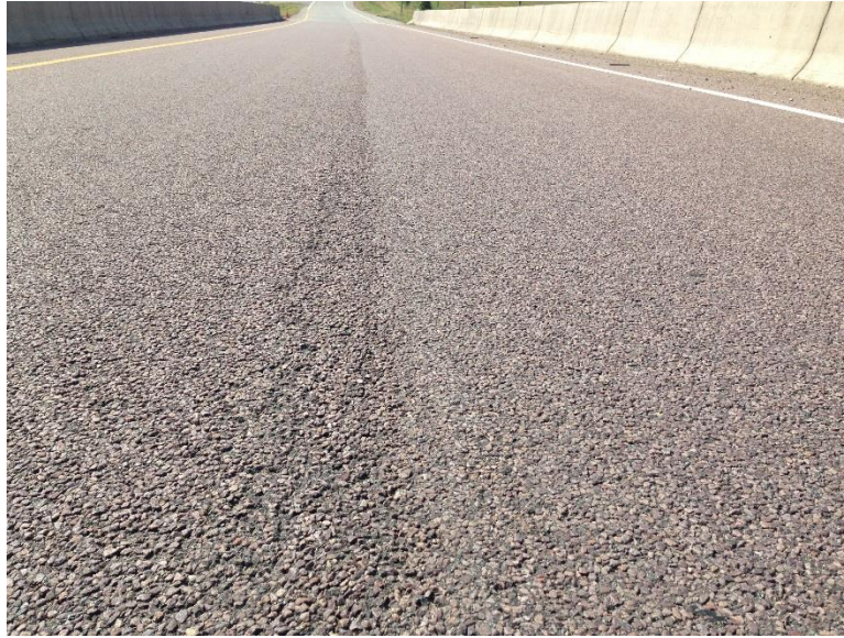
Figure 32: Uneven Snowplow Abrasion due to Uneven Roadway Elevation (Br 86019)
