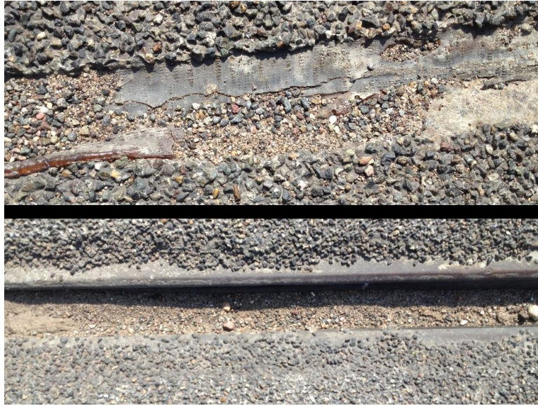
Figure 51: Robert Street (Br 9036) Expansion Joints, Both North (Bottom) and South (Top) of Delamination
