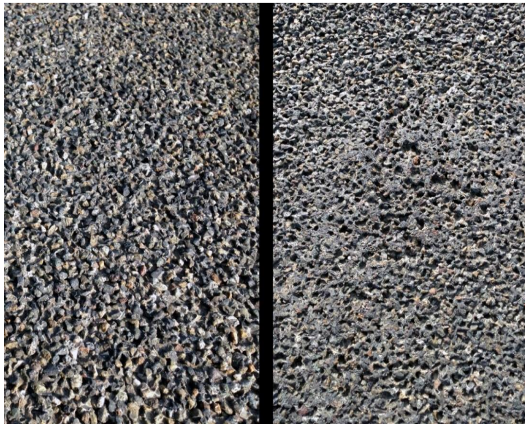
Figure 38: Texture Comparison of Br 4190 (Left: Proper Aggregate Macrotexture, Right: Aggregate Raveling)
