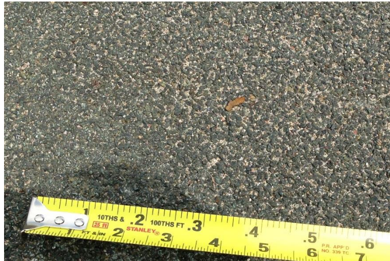
Figure 28: Existing Macrotexture on Bridge 27758
