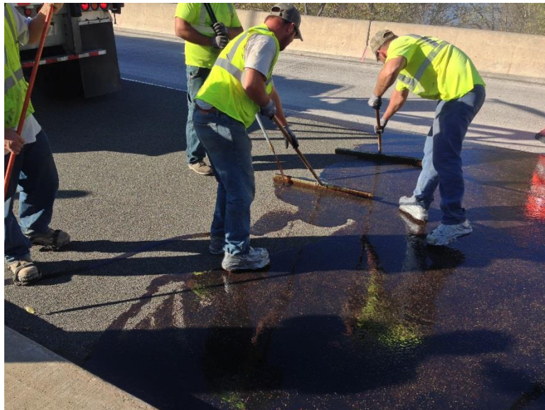
Figure 3: Epoxy is Placed and Levelled
