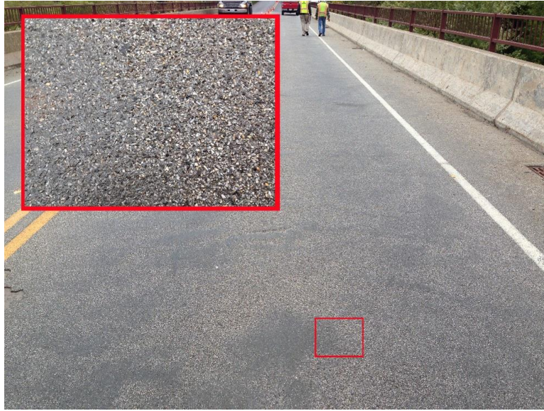
Figure 25: Polished Areas along Bridge 6347
