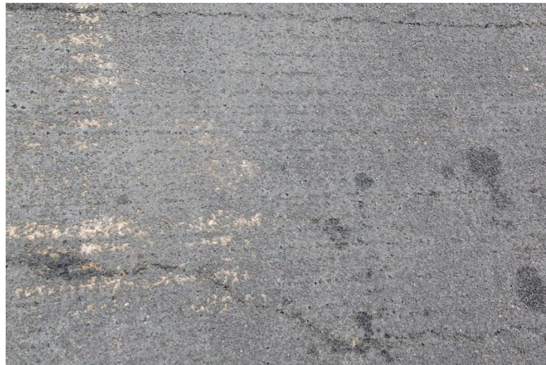
Figure 29: Polished Area on Bridge 27758 along with Transverse Cracks
