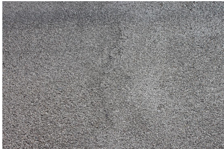
Figure 23: Construction Joint (Bridge 9066)
