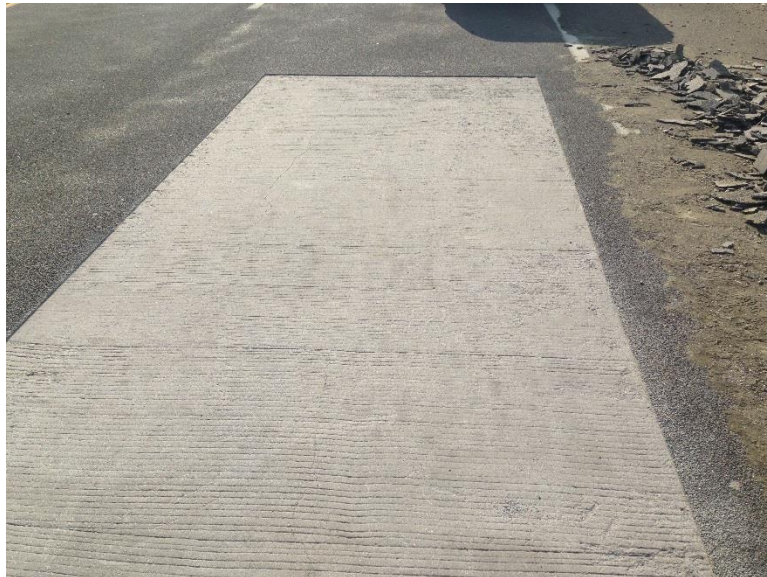
Figure 49: Delaminated Area during Maintenance (Br 4190)
