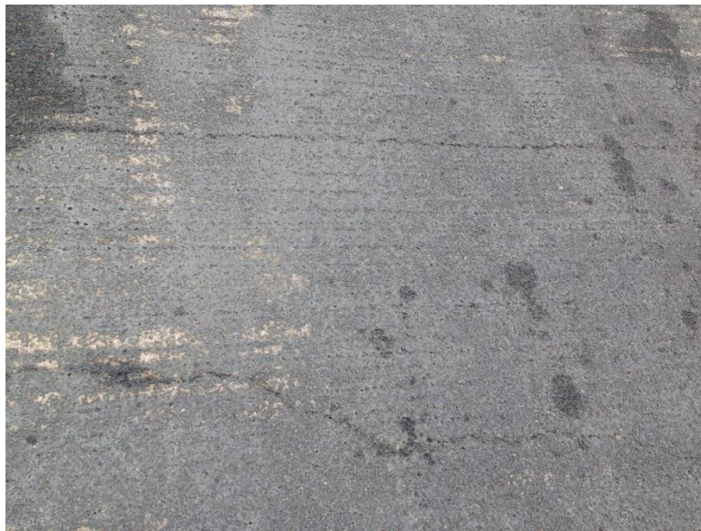
Figure 42: Transverse Cracks on Bridge 27758
