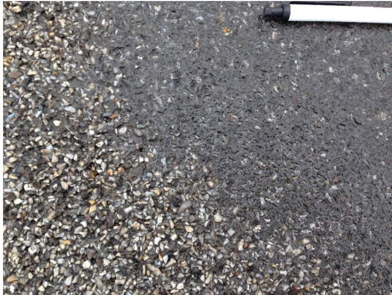
Figure 26: Proper Epoxy Levels (Left Side) Next to Area with Excessive Epoxy (Right Side)
