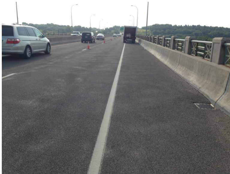
Figure 27: Transverse Snowplow Abrasion (Br 4190)
