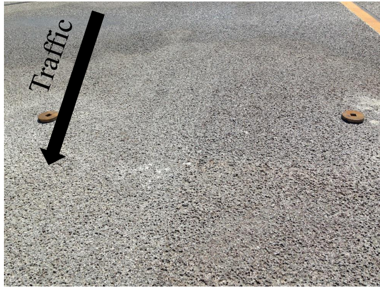
Figure 24: Differences on Both Sides of the Construction Joint (Bridge 14809)
