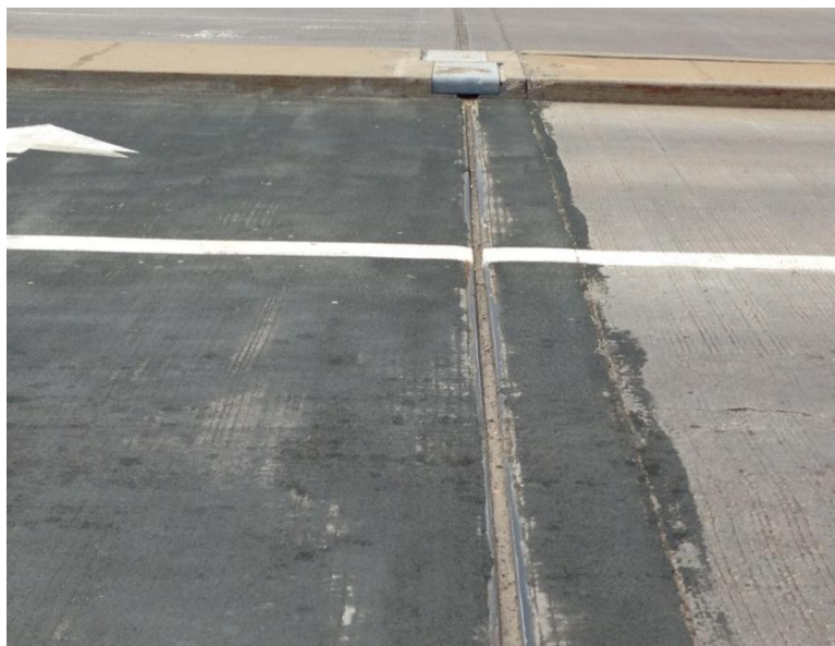
Figure 33: Missing Overlay System near Expansion Joints on Transpo System (Br 27758)
