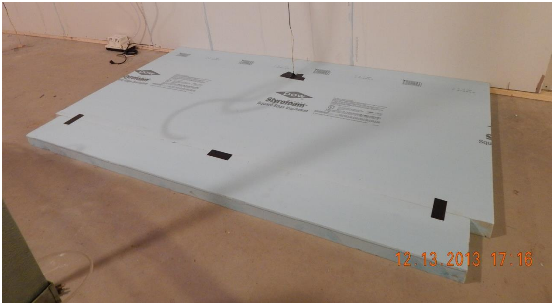
Figure 5-15: Bay 3 Temporary Floor Insulation
