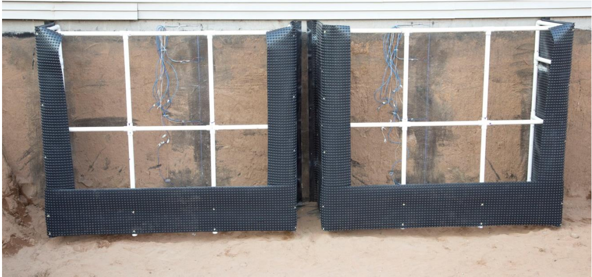
Figure 3-6: Soil Cribs for Soil Containment on Bays 1 and 2
