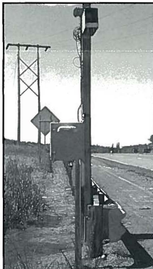
Special video camera housing protects the image from distortions caused by blowing snow, rain, frost, and fog.
