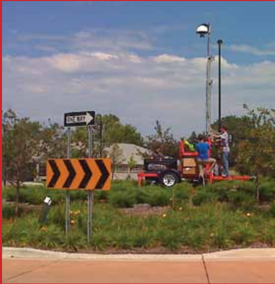
MTO researchers install the system at the test site in Richfield.
