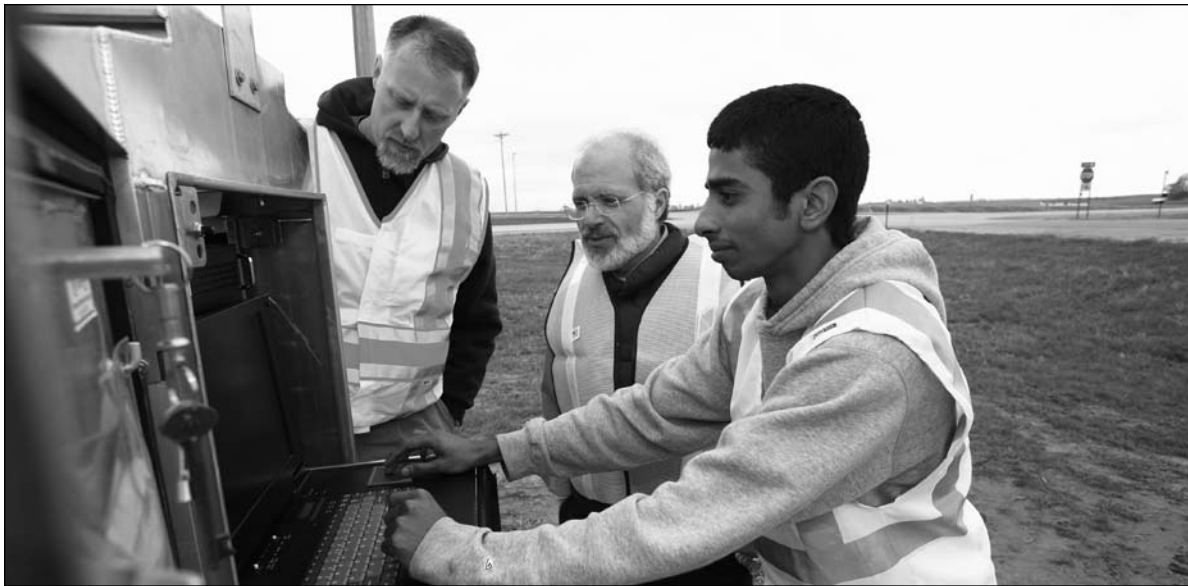
IV Lab director Craig Shankwitz, with Max Donath and Arvind Menon, inspect equipment at Hwy. 52 and Goodhue CSAH 9.
