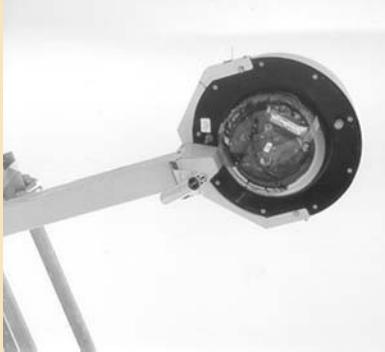
An IRID System sensor mounted on a bridge structure at NATSRL's I-35 research facility
