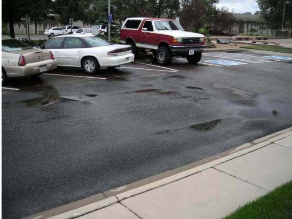
Figure 9.25. Porous asphalt pavement at Denver Waste Management building after a light rain (photo courtesy of K. MacKenzie, UDFCD).
