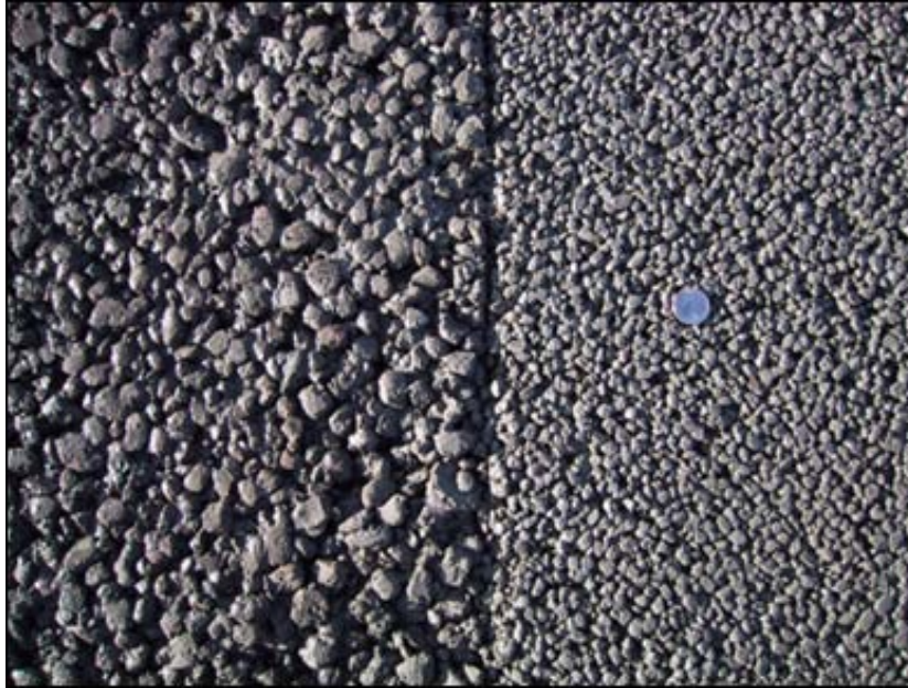
Figure 9.26. Pervious concrete at Lakewood City Shops maintenance building. AASHTO #67 mix is on the left and AASHTO #8 is on the right (UDFCD 2011a). A quarter is placed on the AASHTO #8 pavement for scale.
