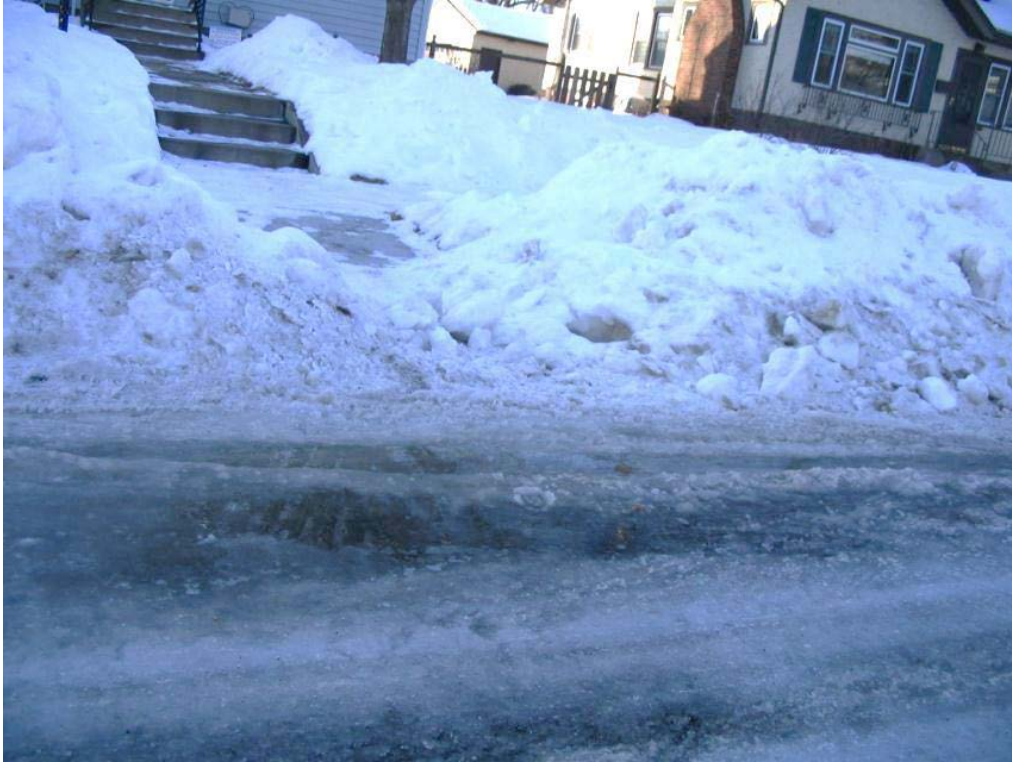
Figure 9.13. Slush gathering and refreezing on the traditional asphalt at Site 1 on January 17, 2010 (Wenck 2014).
