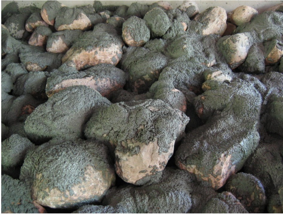
Figure 3.2 - Matrix riprap at Bridge No. 48030, Milaca, MN
