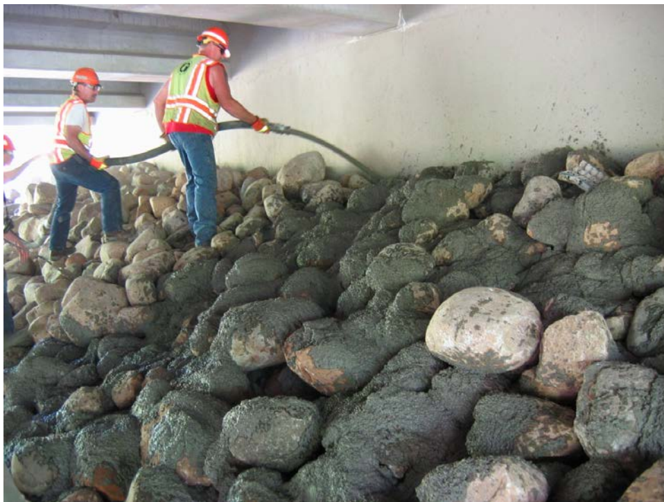
Figure 3.1 -Grout application at Bridge No. 48030, Milaca, MN
