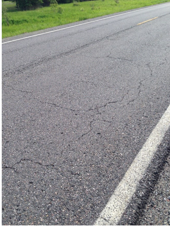
TH 1 good performer-typical crack configuration
