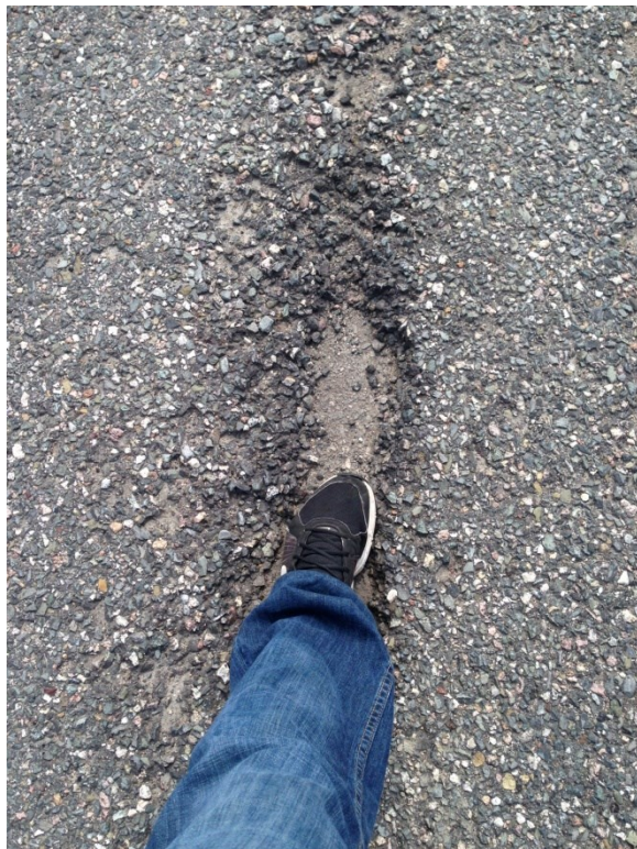
TH 1 poor performer-overlay failure
