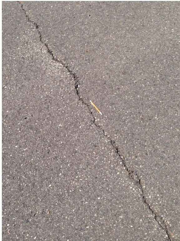
TH 220-typical crack profile
