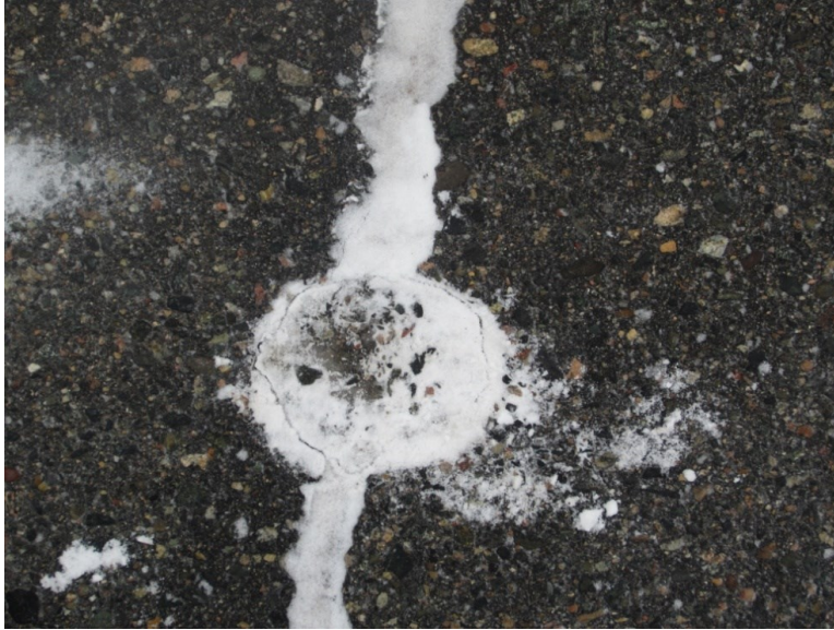
TH 6 good performer-typical crack profile
