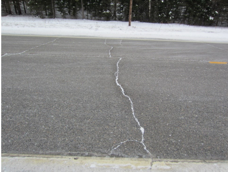
TH 6 poor performer-typical crack configuration
