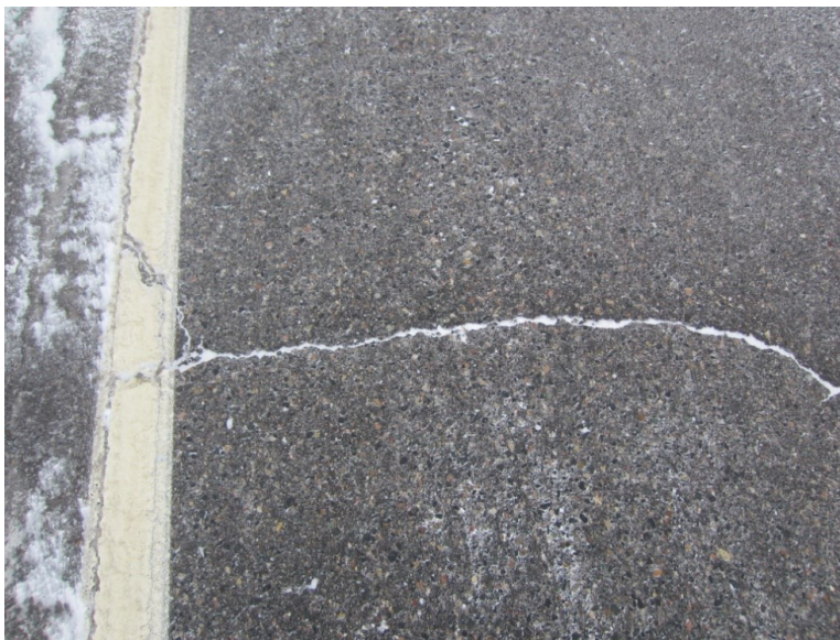
TH 6 poor performer-typical crack profile
