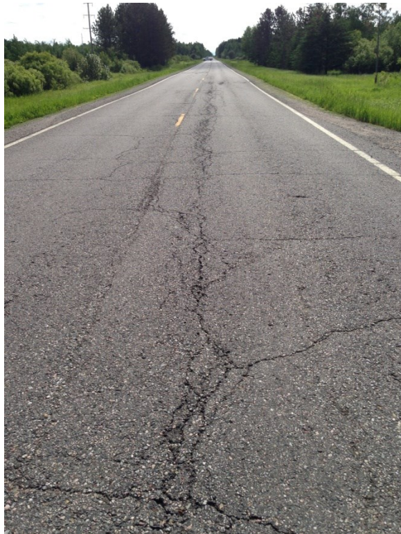
TH 1 poor performer-overview
