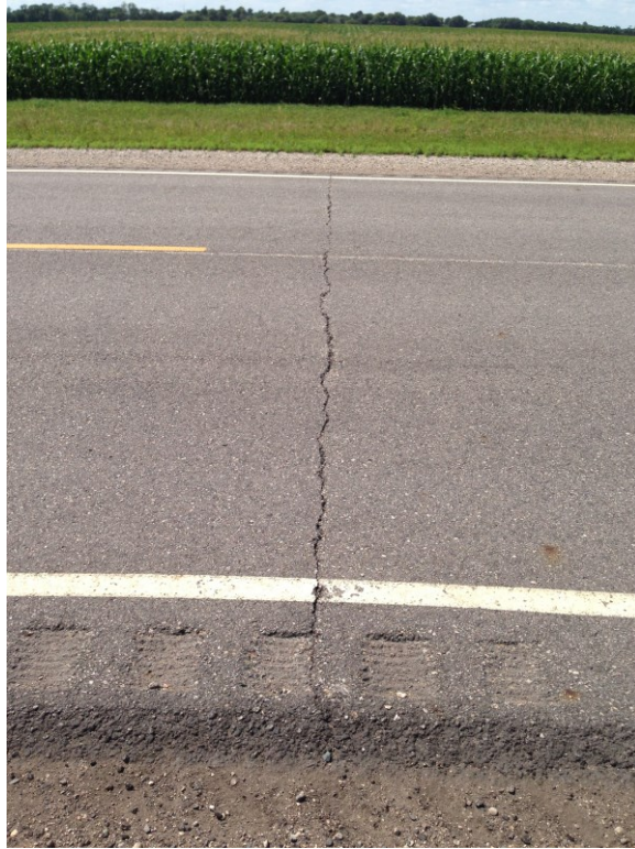
TH 220-typical crack configuration
