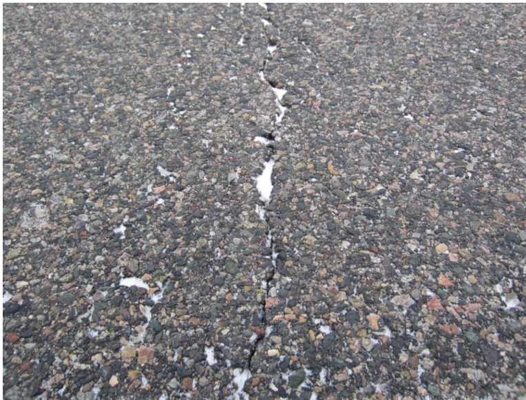
TH 2-typical crack profile
