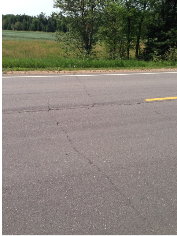
CSAH 10 poor performer: typical crack configuration
