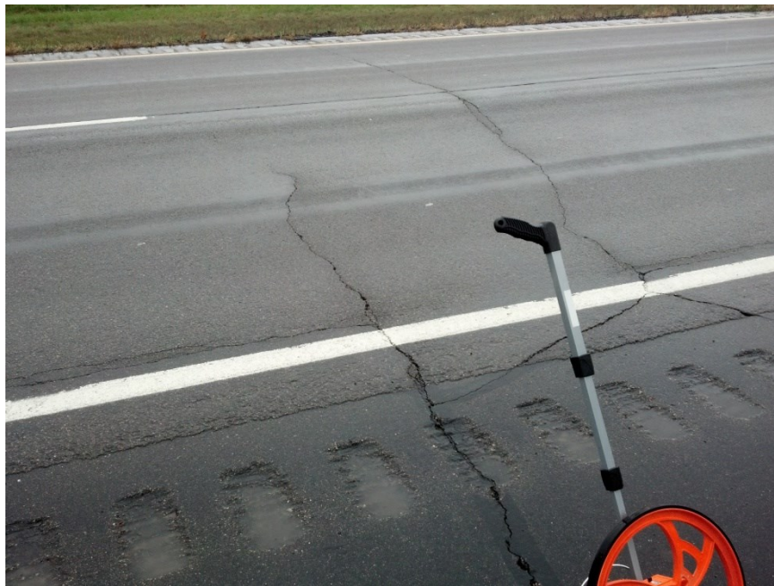
TH 10 good performer-typical crack configuration
