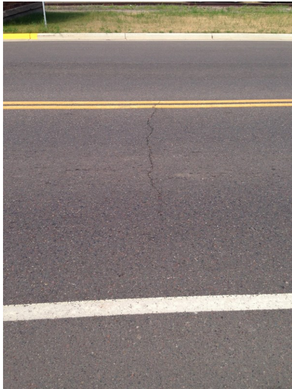
CSAH 30-typical crack profile
