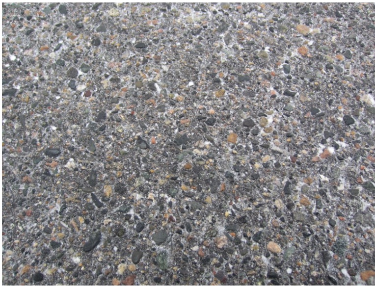
TH 6 poor performer-surface profile
