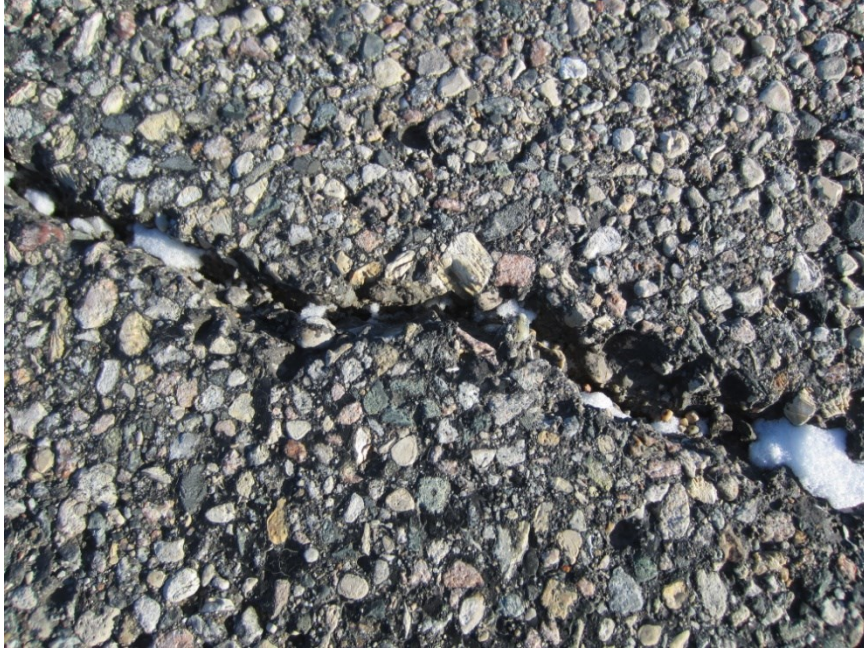
TH 113 good performer-typical crack profile
