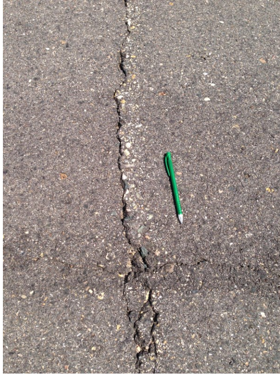
TH 10-typical crack profile
