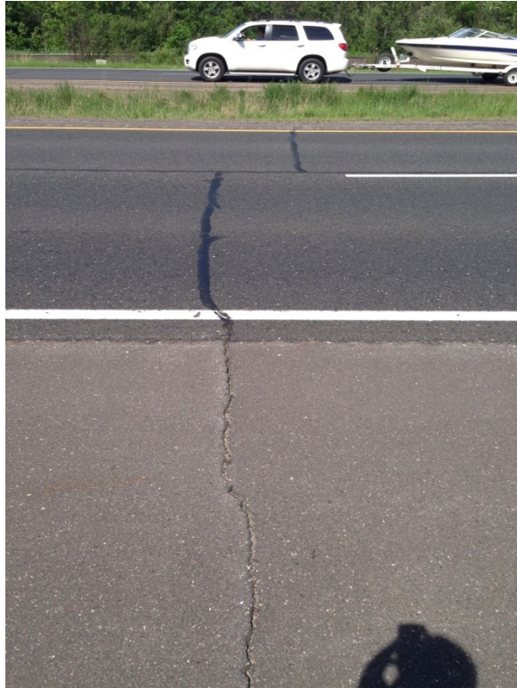
TH 53-typical crack configuration
