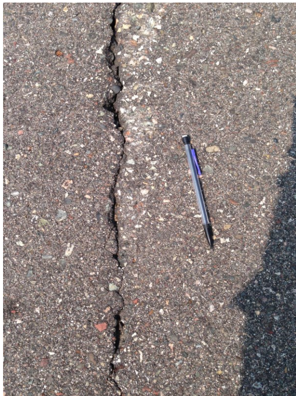
CSAH 10 good performer-typical crack profile
