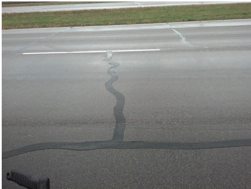
TH 10 poor performer-typical crack configuration
