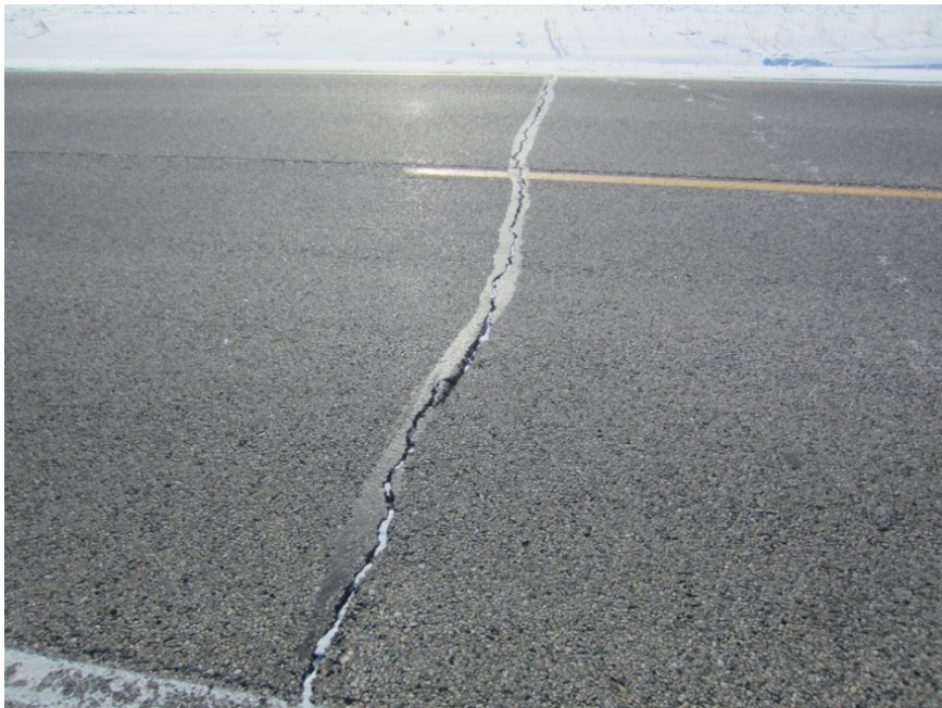
TH 113 good performer-typical crack configuration
