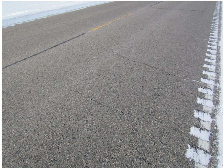
TH 113 poor performer-typical crack configuration
