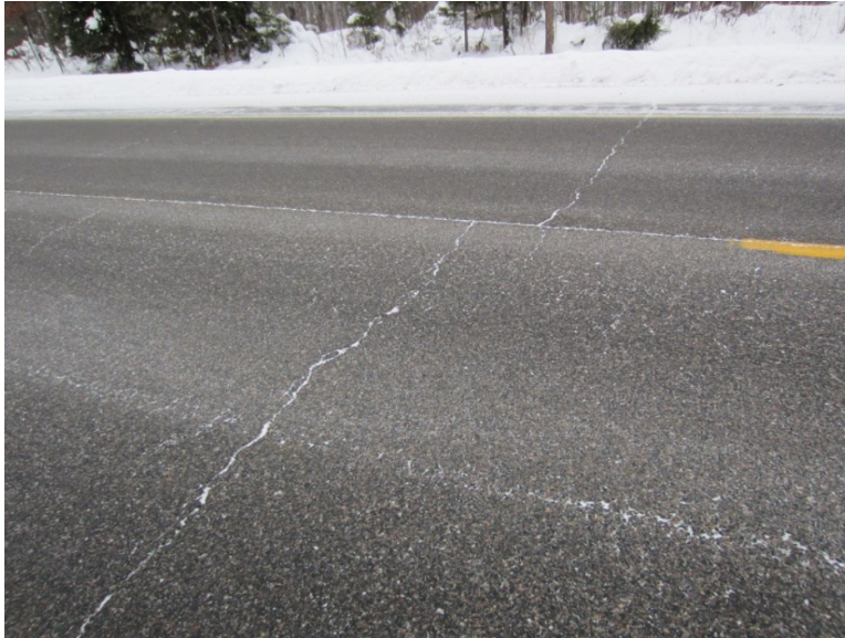
TH 2-typical crack configuration
