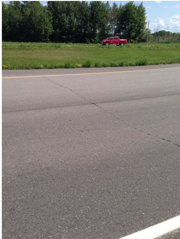
TH 10-typical crack configuration
