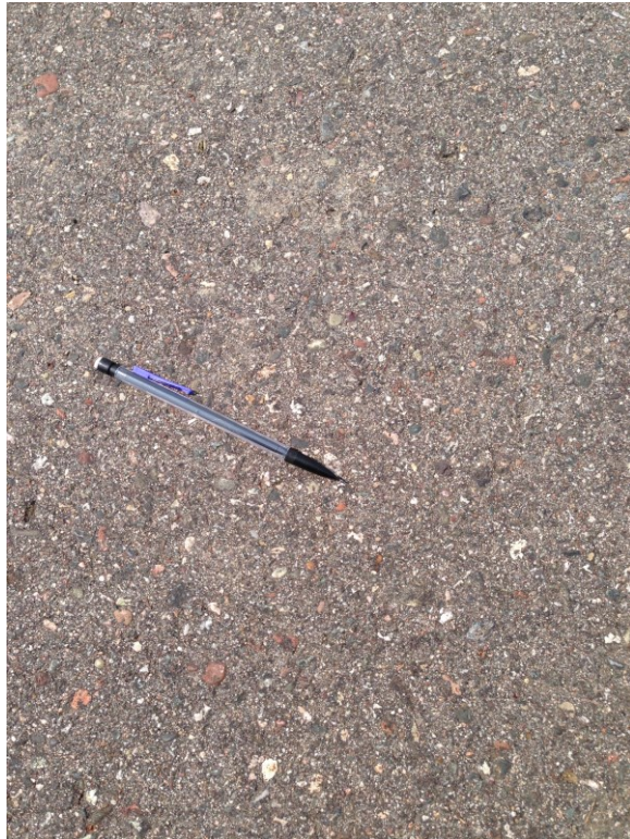
CSAH 10 poor performer-surface profile
