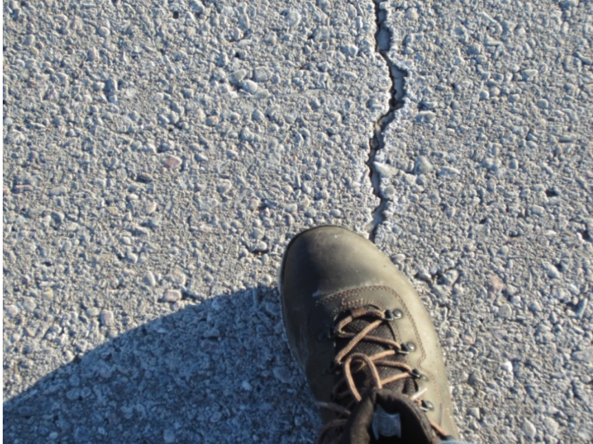
TH 210-typical crack profile
