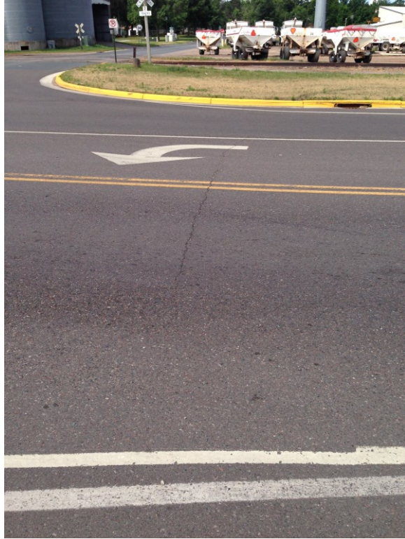
CSAH 30-typical crack configuration
