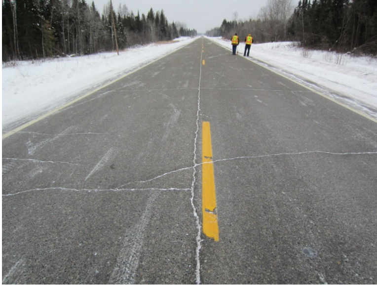
TH 6 poor performer-overview
