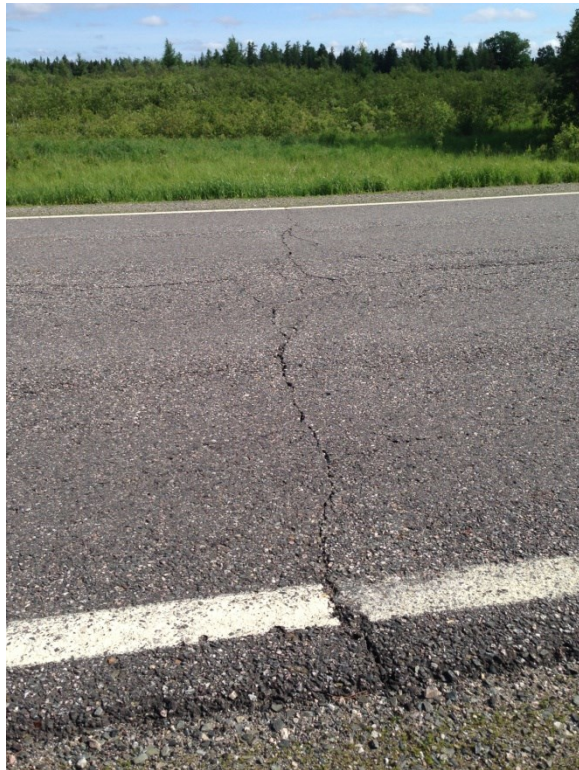
TH 1 poor performer-typical crack configuration
