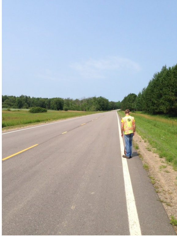
CSAH 10 poor performer-overview
