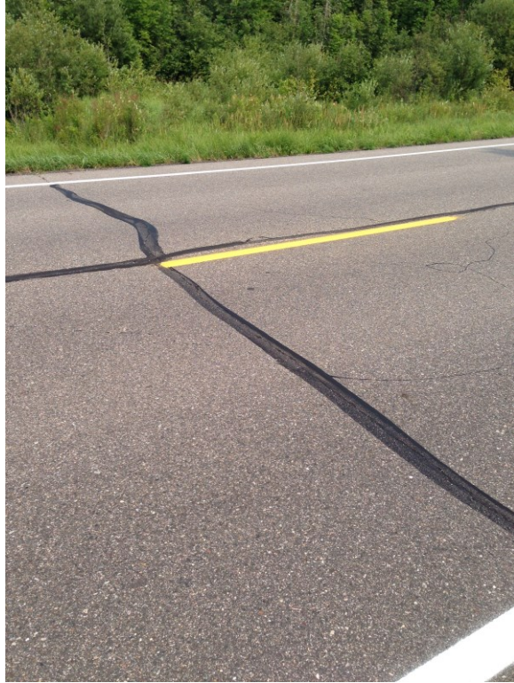
TH 6-typical crack configuration
