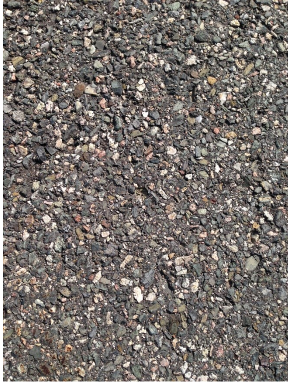
TH 1 poor performer-surface profile
