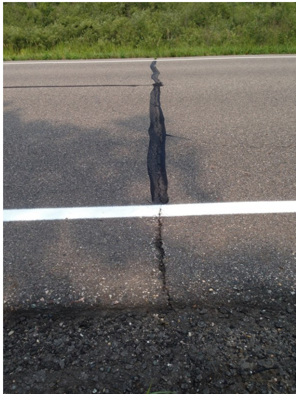
TH 6-typical crack profile
