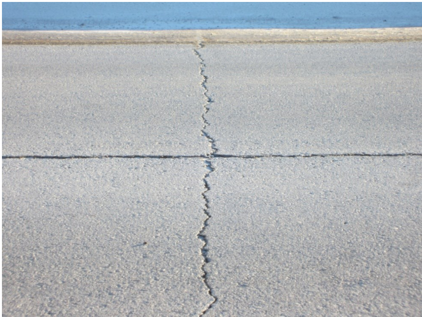
TH 210-typical crack configuration
