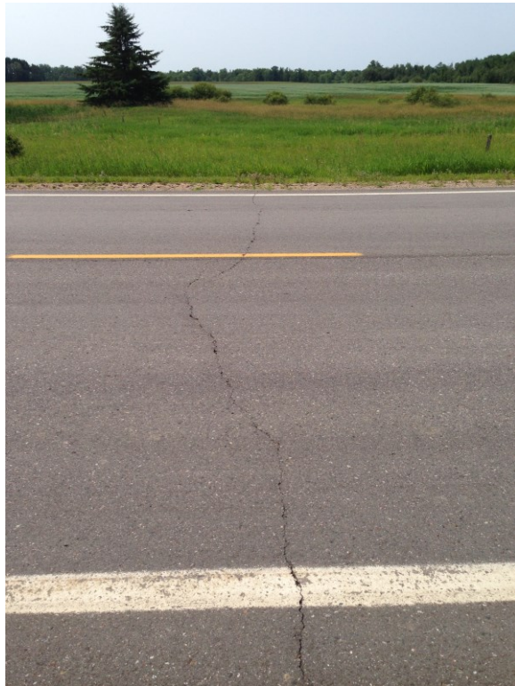
CSAH 10 poor performer-typical crack profile
