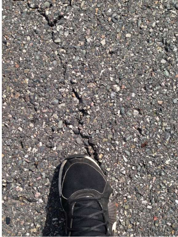
TH 1 poor performer-typical crack profile
