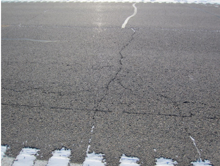
TH 113 poor performer-meandering transverse cracks
