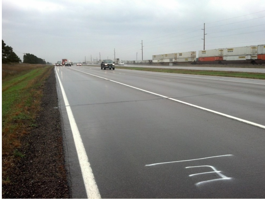
TH 10 poor performer-overview
