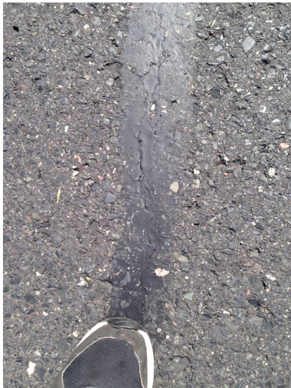
TH 53-typical crack profile
