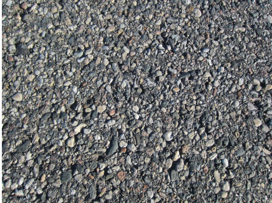
TH 113 poor performer-surface profile
