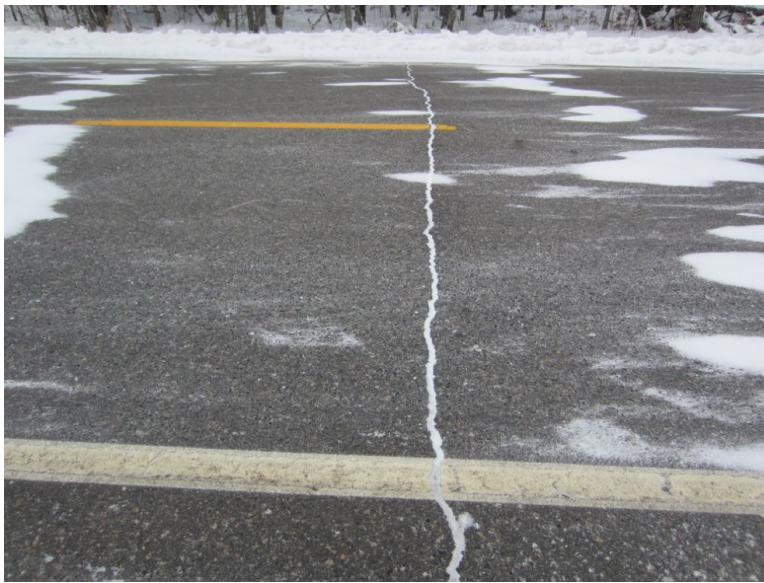
TH 6 good performer: typical crack configuration
