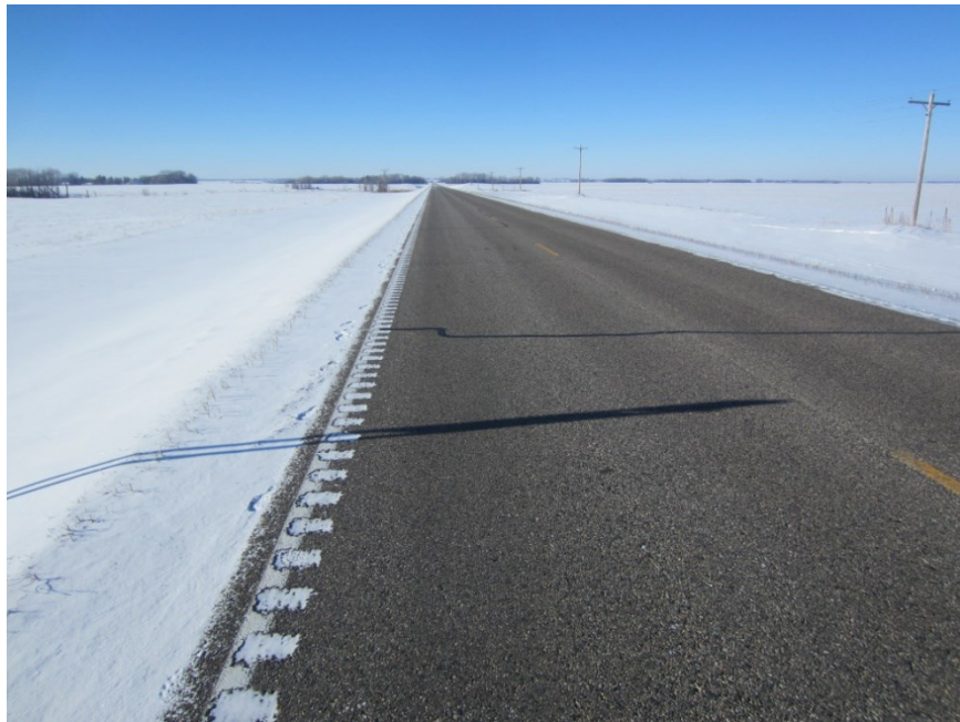
TH 113 poor performer-overview
