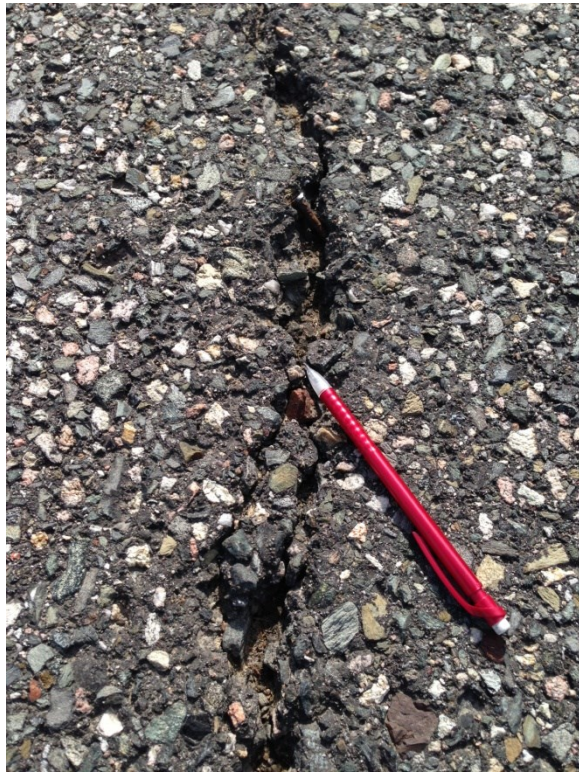
TH 1 good performer-typical crack profile
