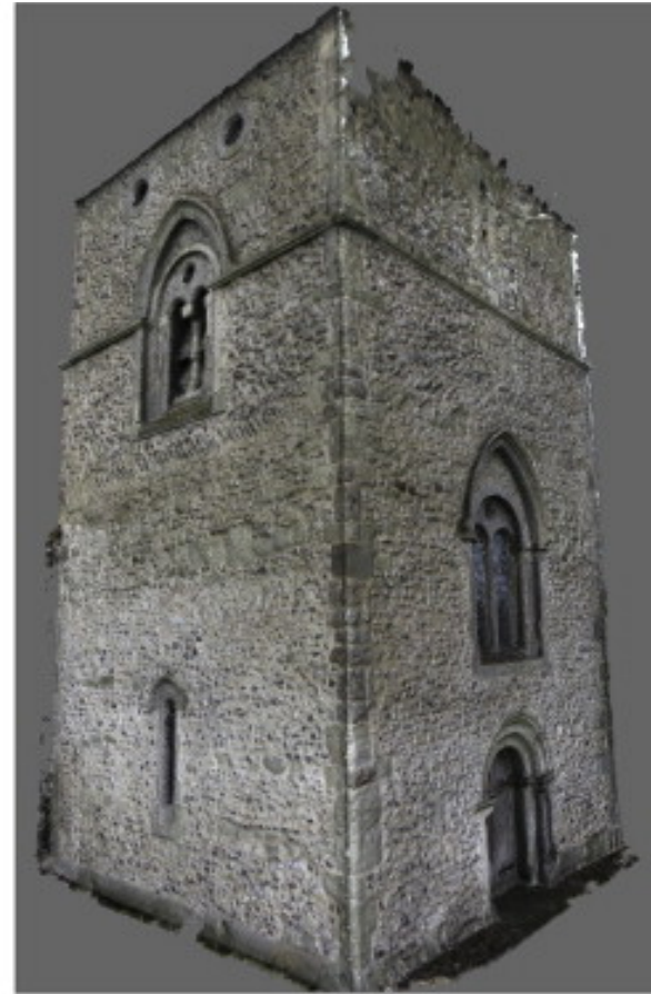
3D point cloud from 244 photos
