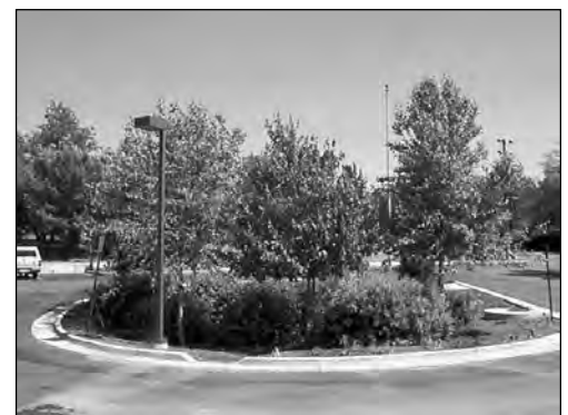
Bioretention parking lot island (Low Impact Development Center)
